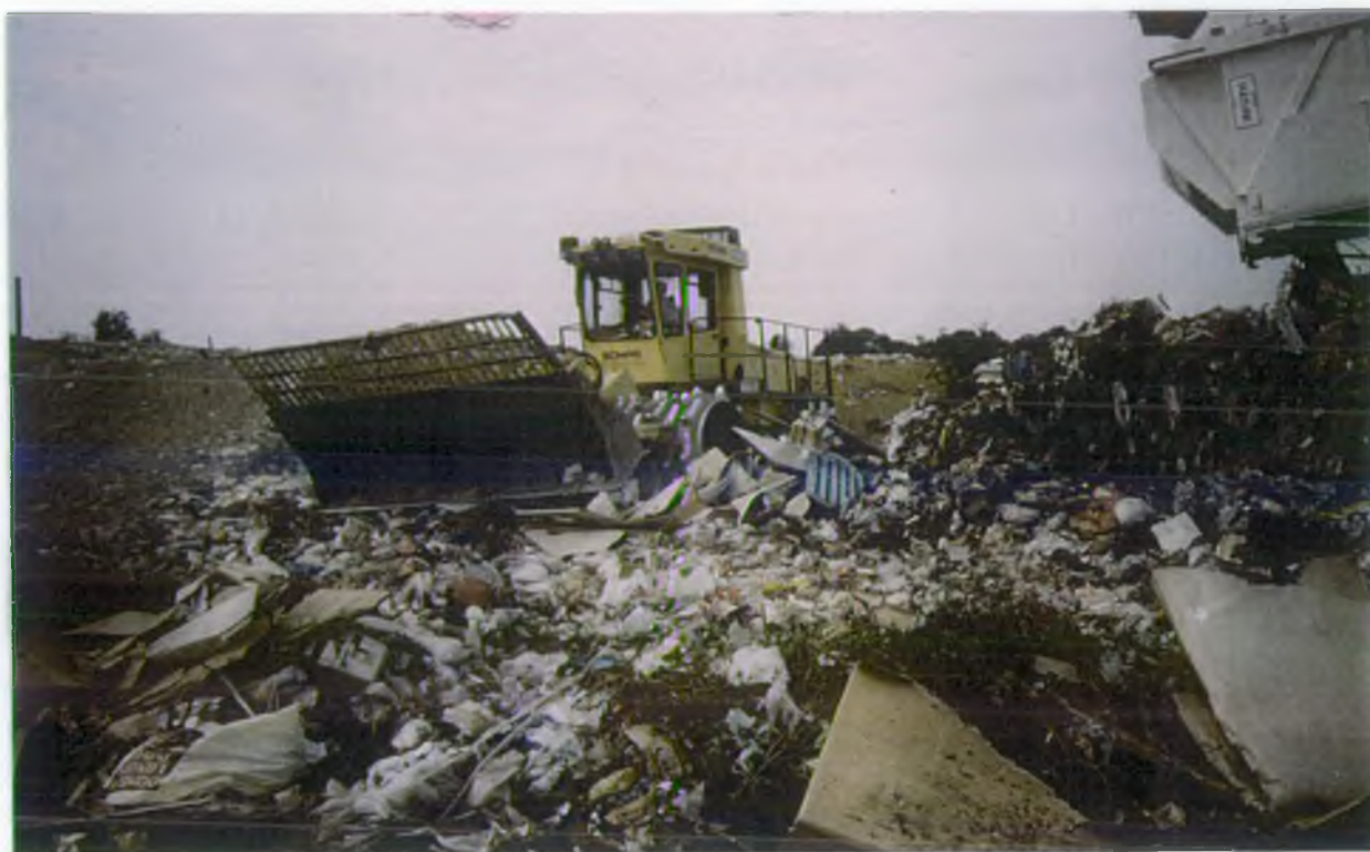
Compaction of waste in a landfill site
