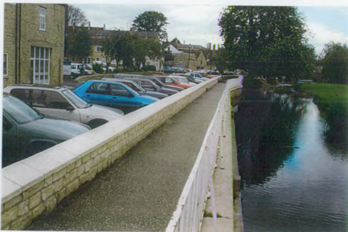
Flood walls at Stamford
