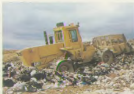
Compacting waste at a landfill site
