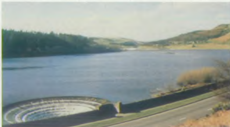
Ladybower Reservoir showing overflow takeoff, Upper Derwent.
