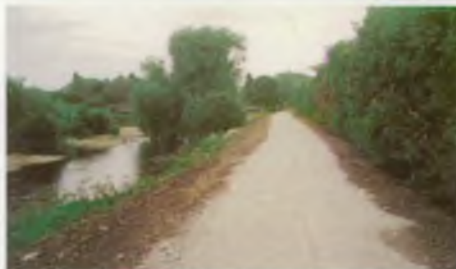
The improved flood bank ends at Raynesway Road Bridge and includes a reinstated cycle path.
