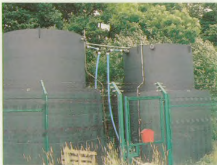
Automated leachate removal system is working round the clock to reduce leachate levels in the site.
