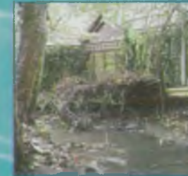
Potential blockage of channel
