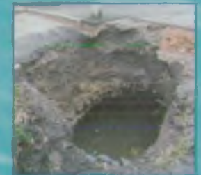
Culvert collapse
