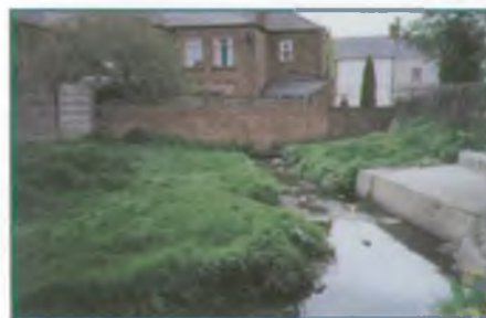
The site for the proposed Edgeworth Drive debris screen
