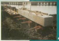
Casting reinforced concrete capping beam to steel sheet pile wall.
