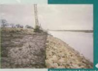
Stone revetment being replaced using a 22RB dragline to protect batters from erosion on tidal channels.
