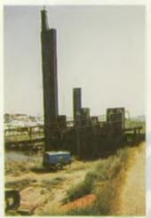
Driving steel sheets plies to farm cofferdoms, cut off walls etc.
