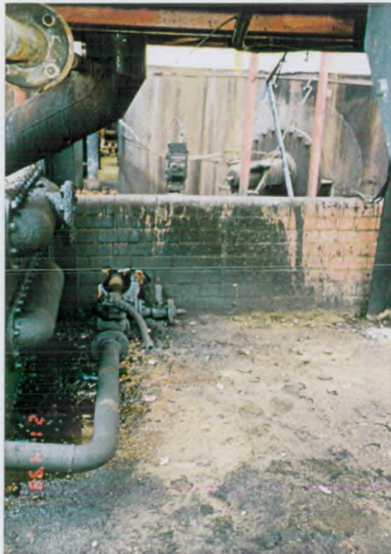
PHOTOGRAPH REF SW/0169/013: BULK TREATMENT PLANT - DAMAGED BUNDING
