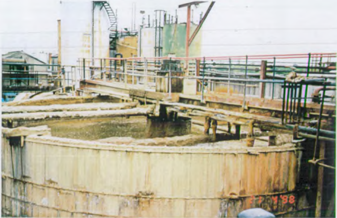
PHOTOGRAPH REF SW/0169/013: BULK TREATMENT PLANT - DAMAGED BUNDING
