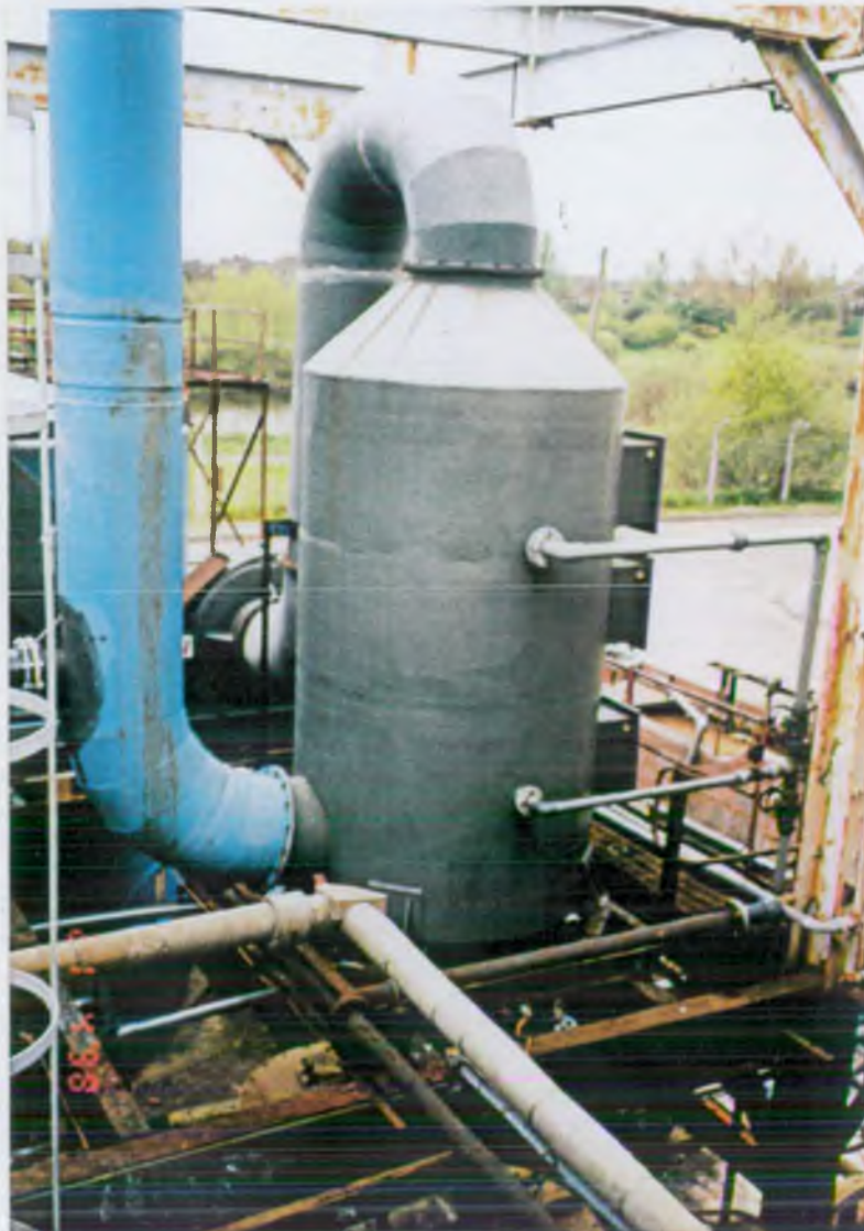
PHOTOGRAPH REF SW/0169/011: BULK TREATMENT PLANT - CAUSTIC SCRUBBER
