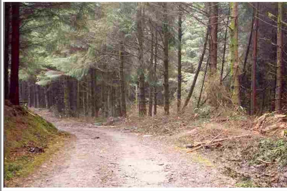
**Plate 3.4 Brash relief road running parallel to stone-surfaced forest road**
