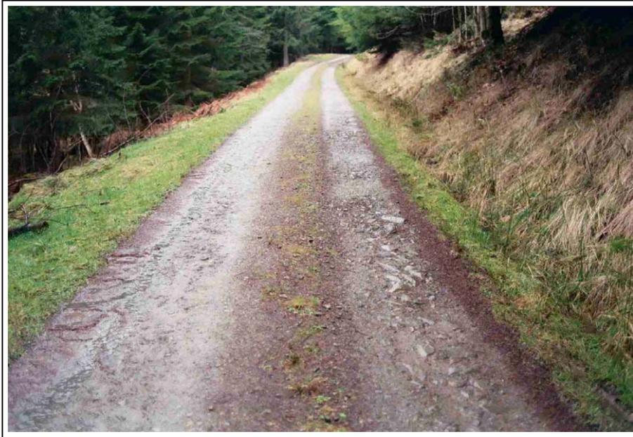
**Plate 3.18 Stone-surfaced track providing for heavy access by forwarders and timber wagons**
