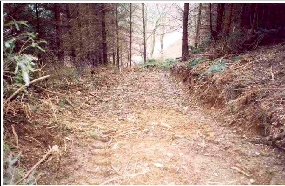
**Plate 3.15 Excavator grading of side slope to provide skidder access**
