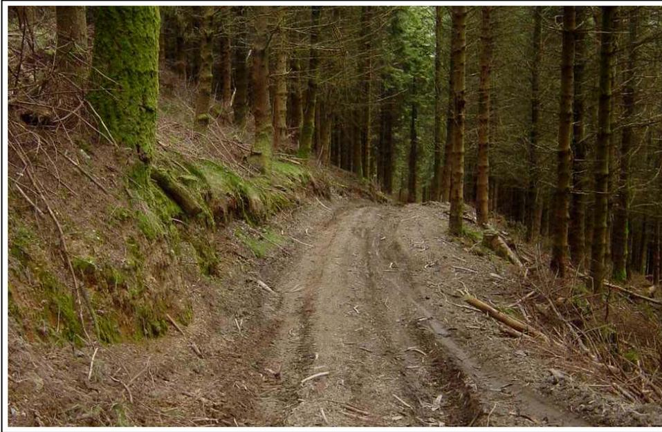
**Plate 3.11 Unsurfaced track beginning to show signs of rutting**
