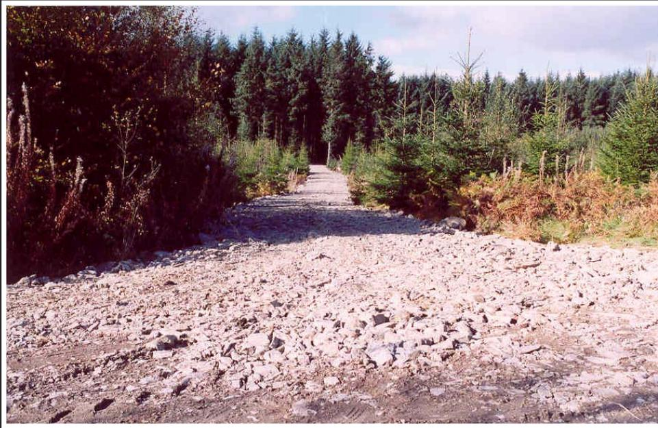
**Plate 3.7 Newly constructed stone-surfaced access track connecting the existing forest road (foreground) to the forest rack network**
