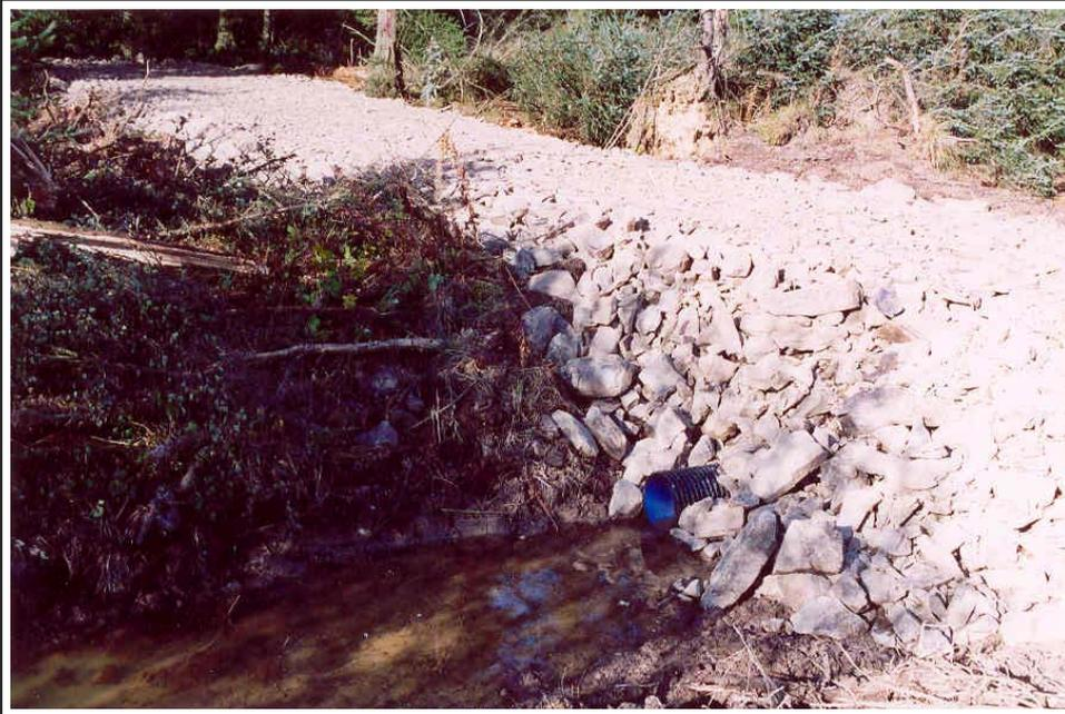
**Plate 3.9 Culvert instated as part of new track construction at Clocaenog Forest**
