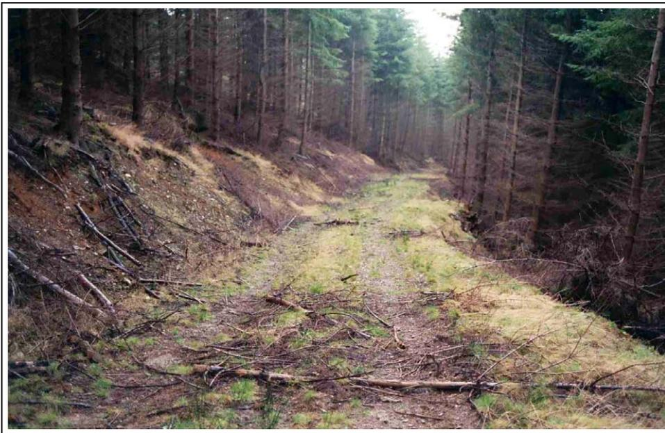
**Plate 3.17 Unsurfaced access track constructed to allow machine access for timber extraction during transformation thinning**
