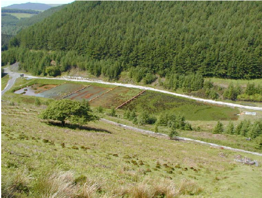
Figure 1.5 Photograph looking down on the Garth Tonmawr system with the minewater entering the system on the right.
