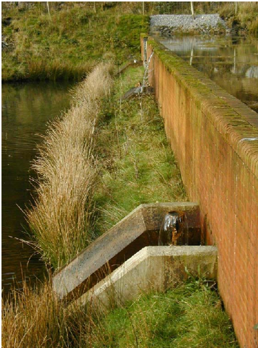
Figure 3.3 Flow pathways over and through cell 2 of the Garth Tonmawr system.
