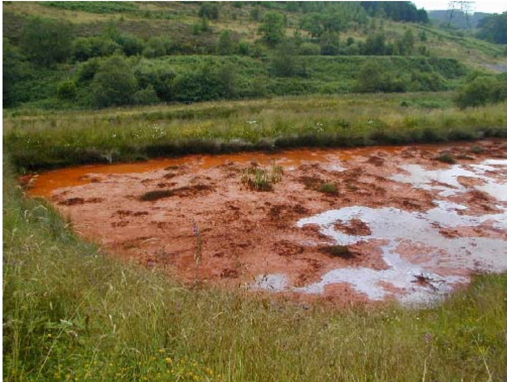
Figure 3.8 Iron oxide and hydroxide accumulation on the surface of the Whitworth A RAPS.
