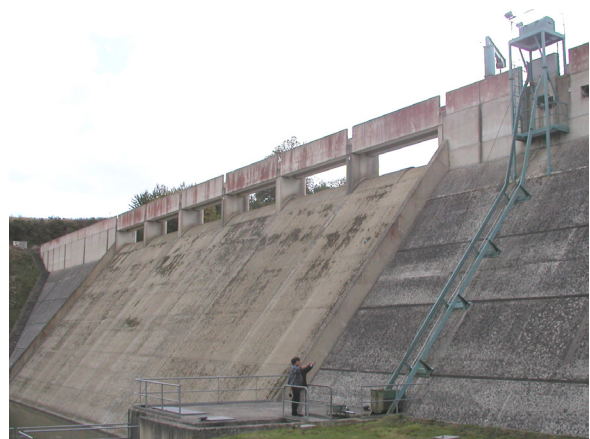
Figure 4.3.7. Eel lift at Bois Joli Dam.
