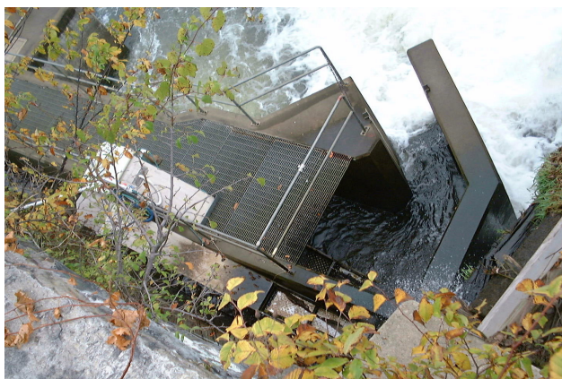
Figure 4.4.15. Eel pass-trap at Westfield Dam viewed from above. The eel pass is the pale grey installation on top of the Denil fish pass. The eel pass has two ramps, one collecting fish from within the fish pass, the other from between the fish pass and the dam wall.
