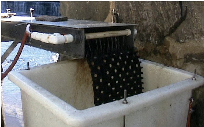
Figure 4.4.14. Akwadrain substrate extending beyond top of ramp at Greenville Dam eel pass. Photo A Haro
