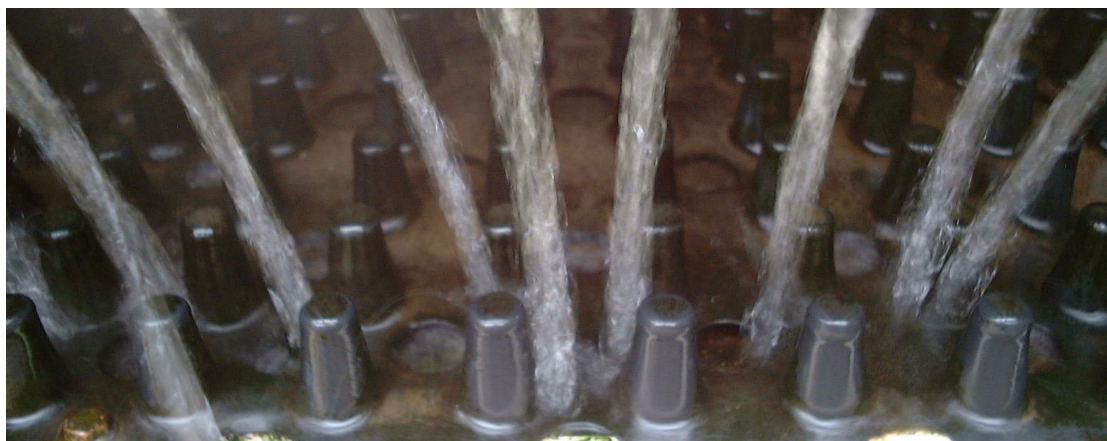
Figure 4.4.16 Top of one of the ramps at the Westfield pass-trap showing the Akwadrain substrate and the jets of water irrigating the ramp.
