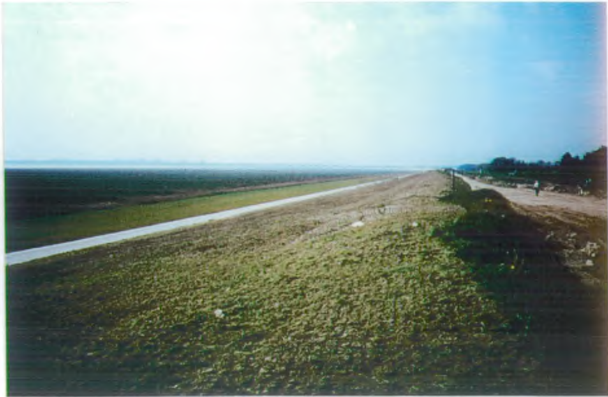
15. A section of reconstructed dike (looking seaward) at Cäciliengroden
