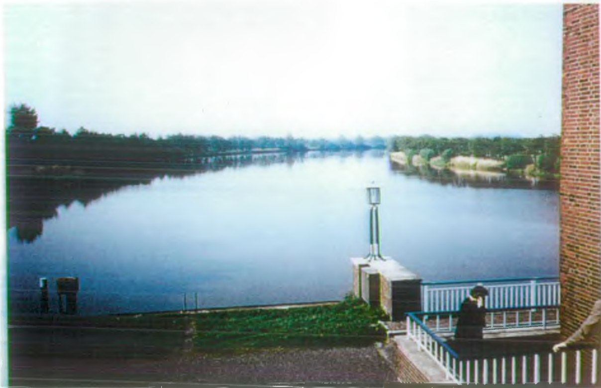
12. Storage basin upstream of drainage sluice at Dangast
