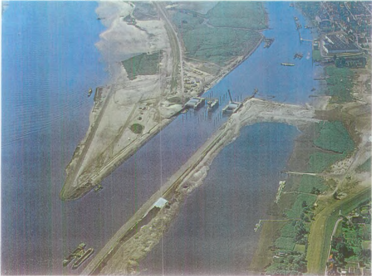
The Hunte Storm Surge Barrier
