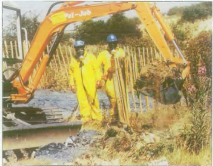
FIGURE 2: REMOVAL OF CYANIDE DURING REMEDIAL WORKS.
