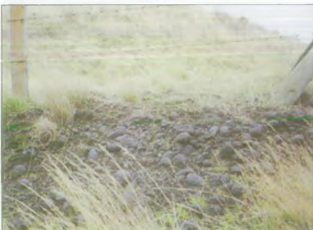
FIGURE 11: SMELTING WASTE BRIQUETTES - USED TO RAISE BANKS ON PARTS OF THE SITE.
