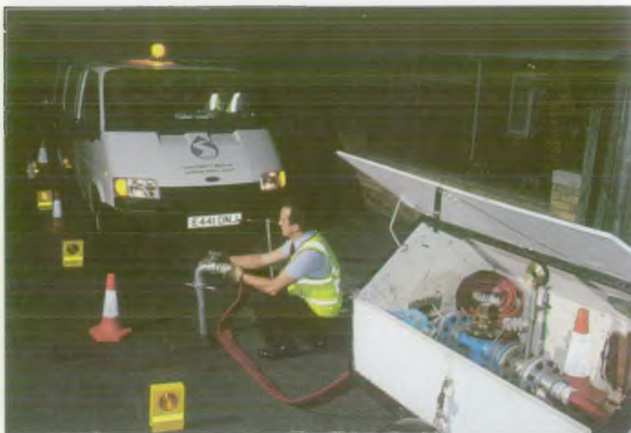
Water Company repairing leaking main.
