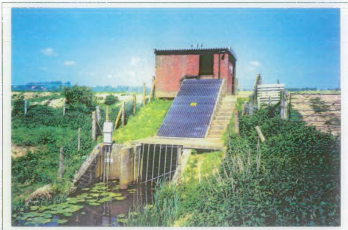
Court Lodge Pumping Station - Southern Region Archimedean Screw Pump Installation
