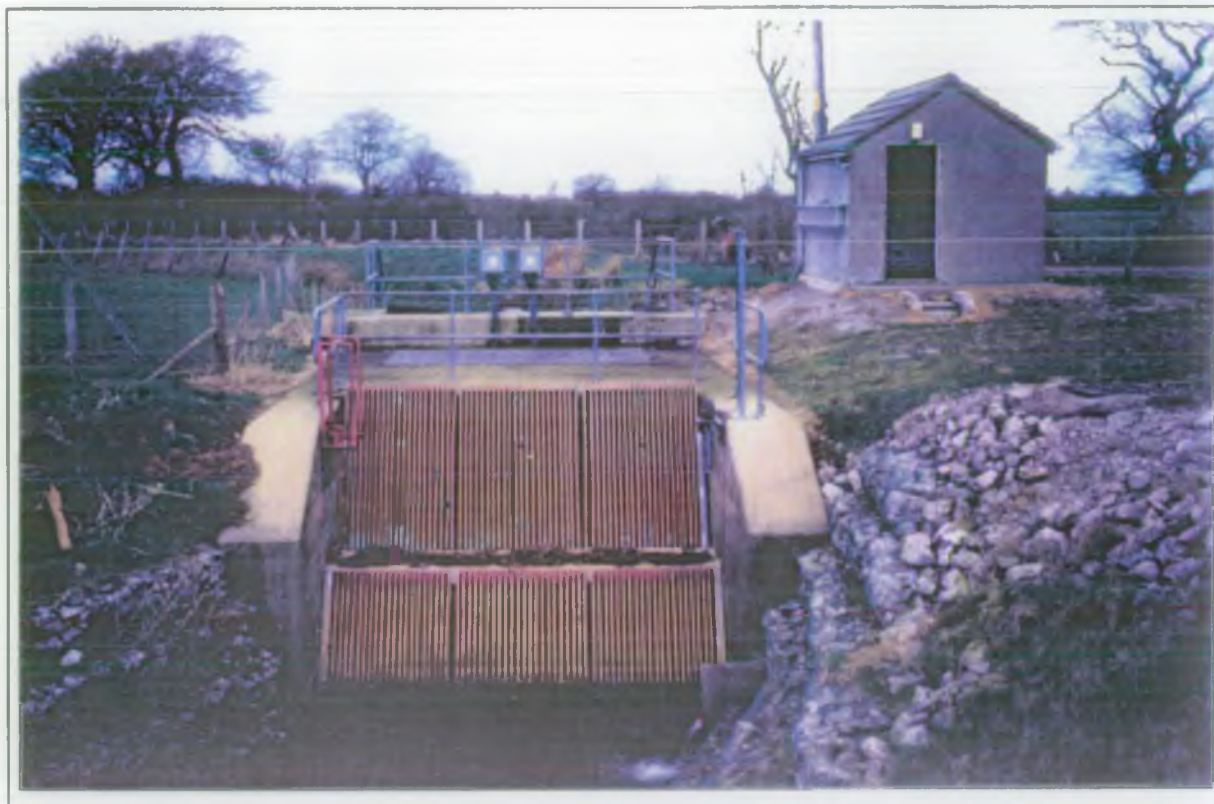
Wolsty Pumping Station - North West Region Submersible Pump Installation Capacity 0.80 cumecs
