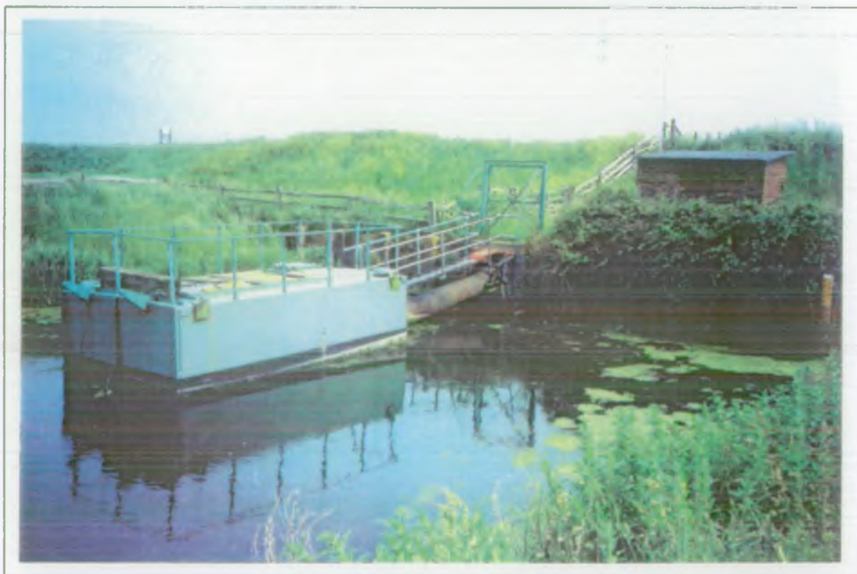
Rodmell Pumping Station - Southern Region Floating Pump Installation
