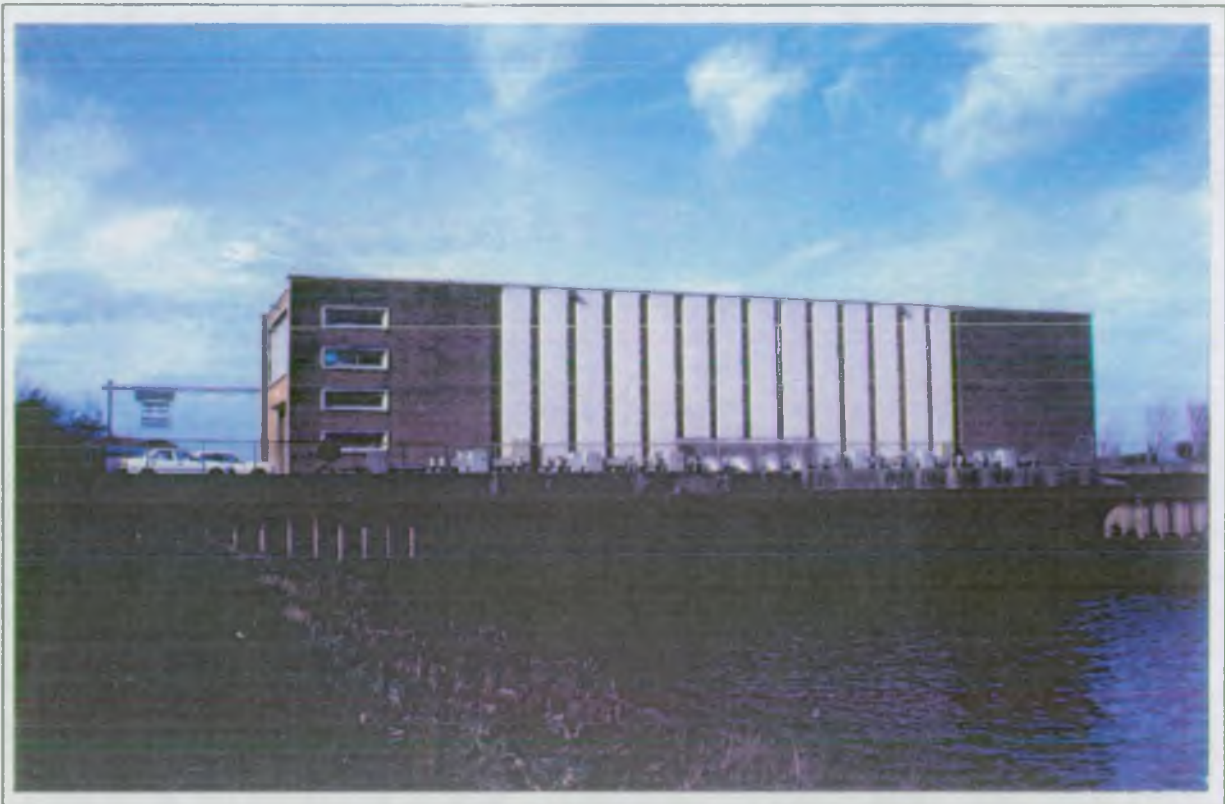
Altmouth Pumping Station - North West Region Axial Flow Vertical Lift Station Capacity 84 cumecs
