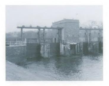
result of high tides, which regularly exceed the Chester weir crest level. Accompanying these flow reversals there are temporary variations in river levels of a metre or more over 12 hours. These unsteady hydraulic conditions cause problems for hydrometric measurement, real time control of regulation releases and prediction of times of travel within the reach.
