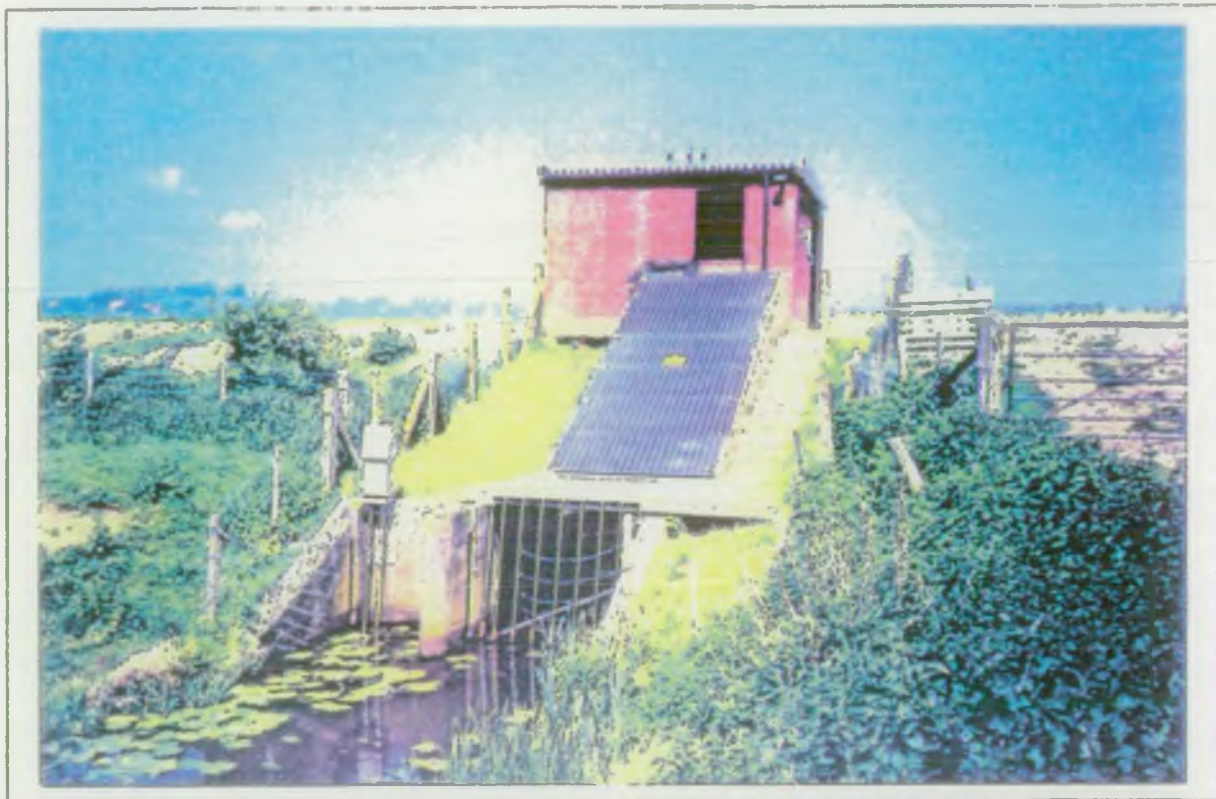
Court Lodge Pumping Station - Southern Region Archimedeon Screw Pump Installation
