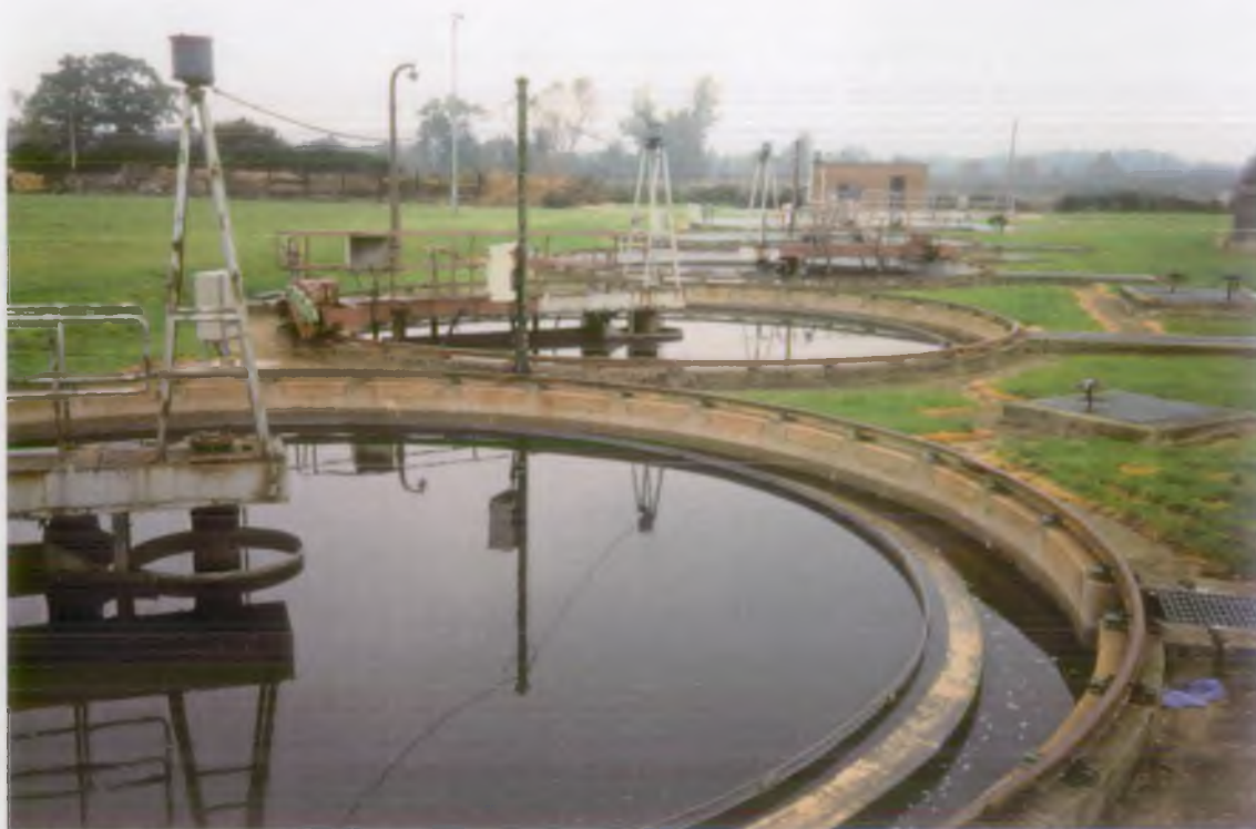
Old Final Settlement Tanks (Humus Tanks)
