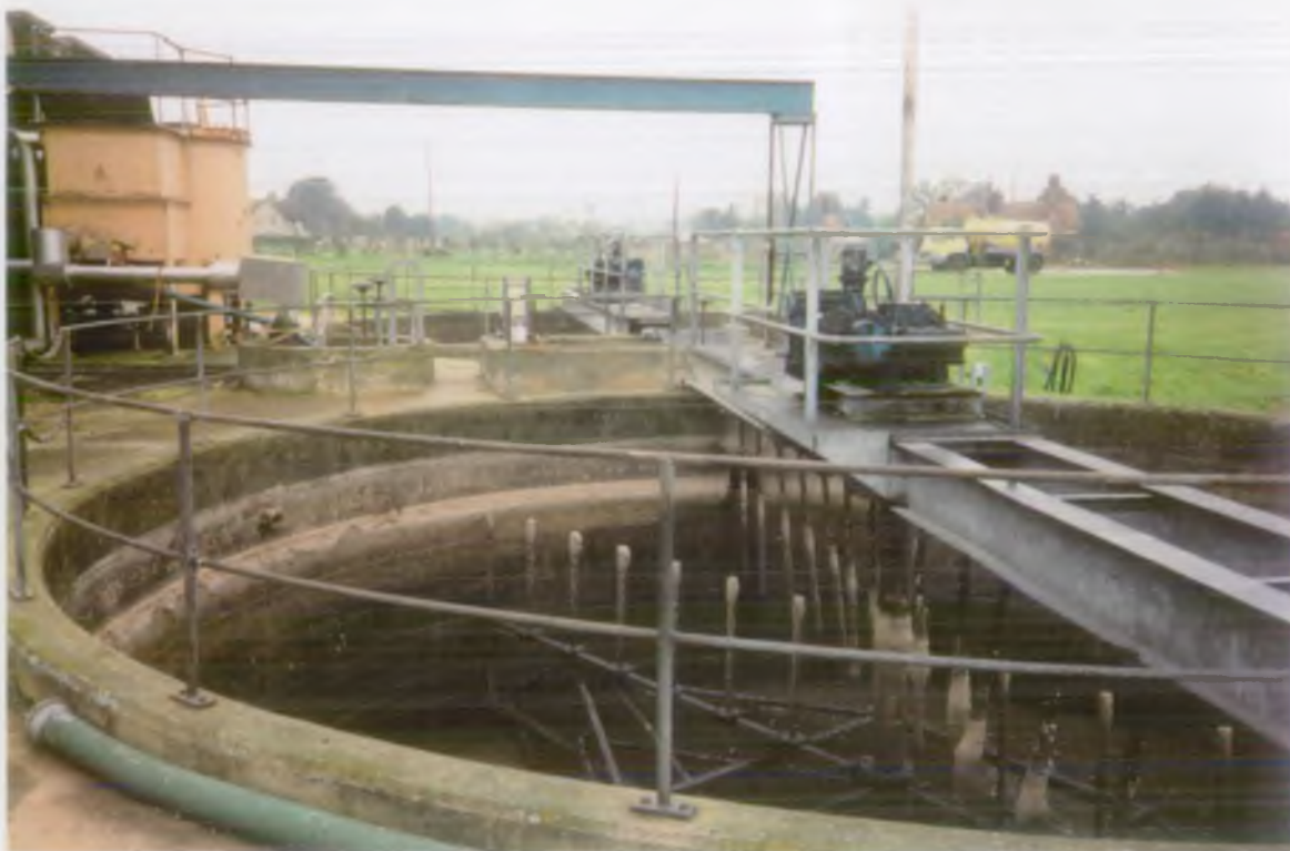
Sludge Holding Tanks
