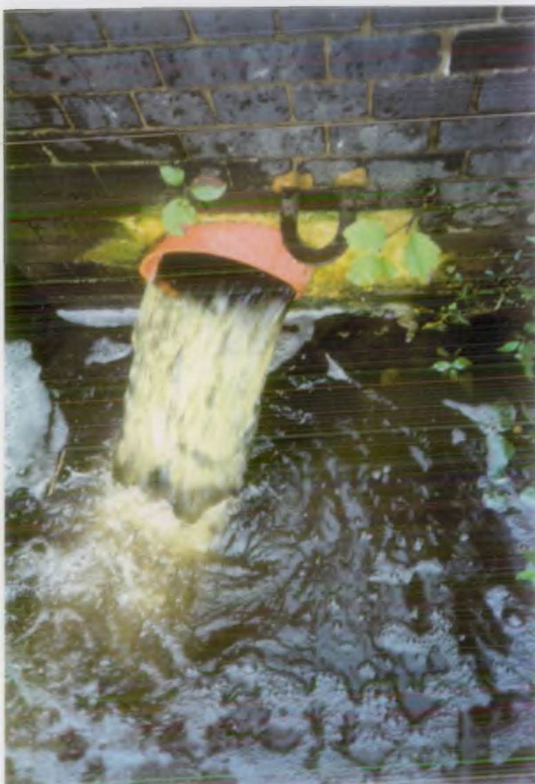
Godalming STW No. 2 outfall. No. 3 outfall below but submerged. Discharge from land drain serving land Treatment Area.
