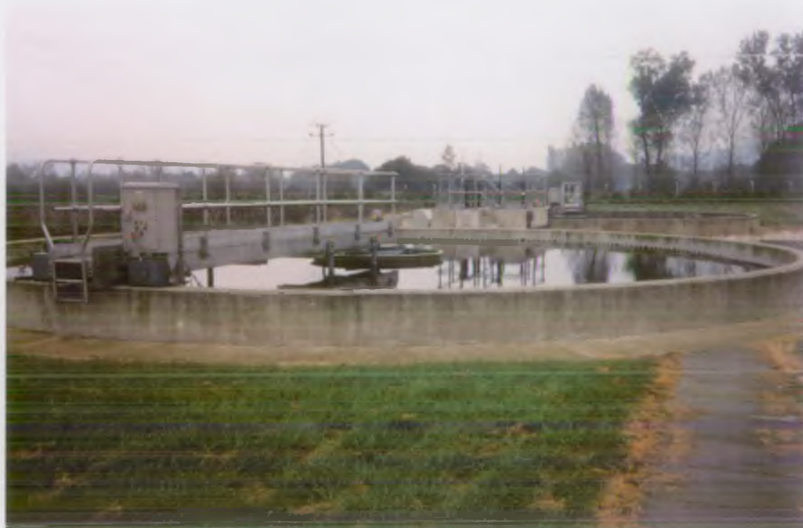
New Final Settlement Tanks (Humus Tanks)
