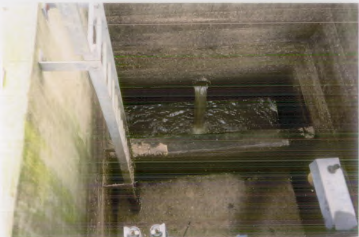
Press House Liquor return chamber (adjacent to Final Effluent Chamber shown above)
