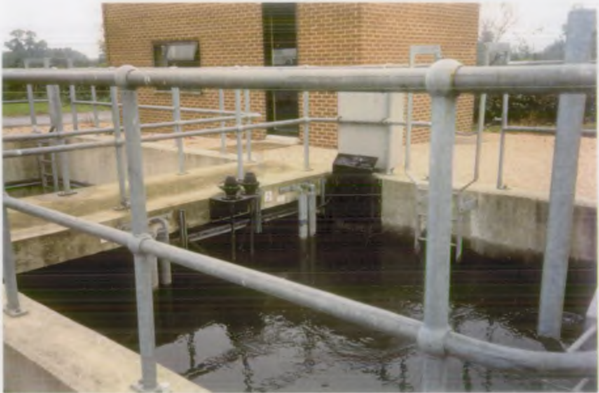
Final Effluent Chamber and Pump House (recirculation)
