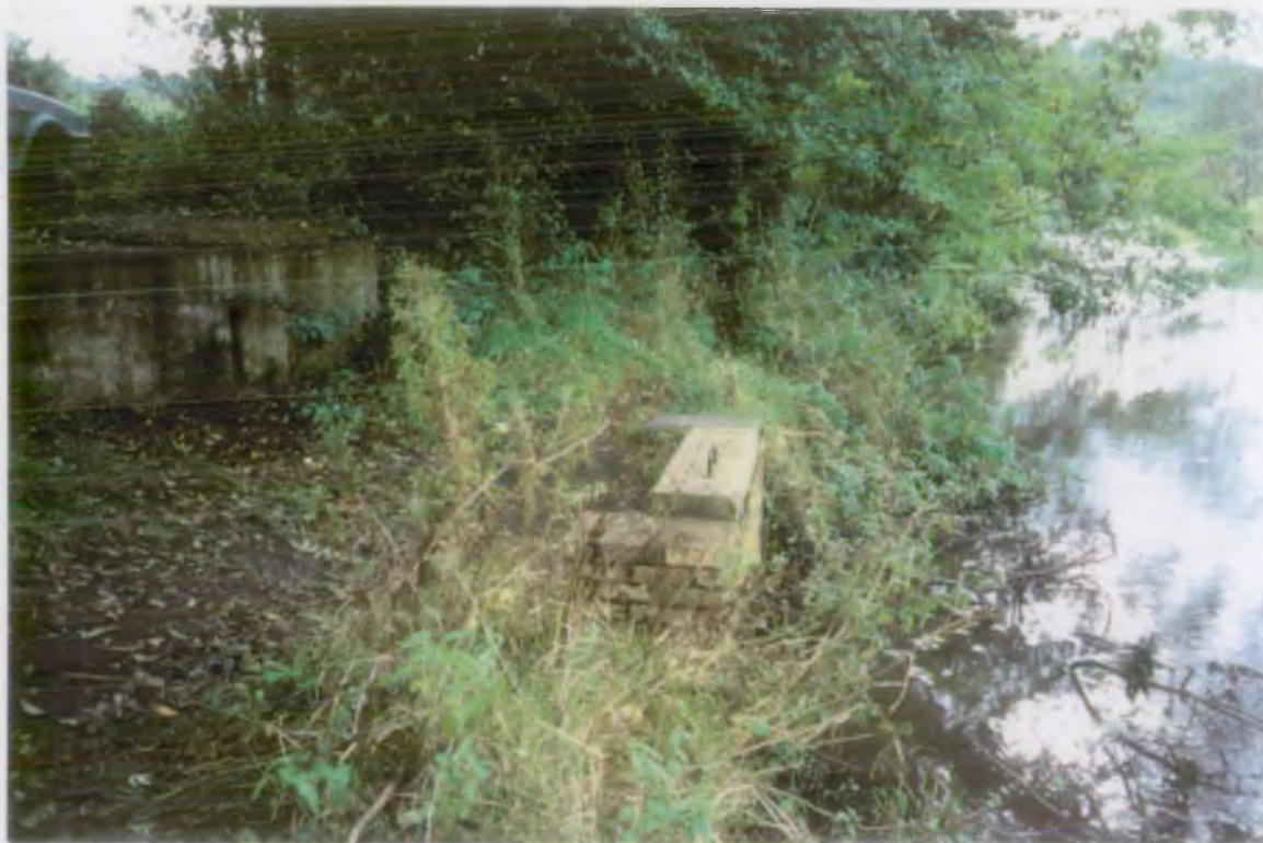
Godalming STW No. 1 outlet to R. Wey (Direct discharge from Final Effluent Chamber)
