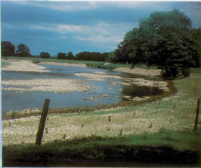
13. Newly planted willow stakes. Willow kidding has been carried out to protect the bank toe. Notice the gentle gradient of the reprofiled bank. The area has also been sown with grass seed to protect the soil surface.
