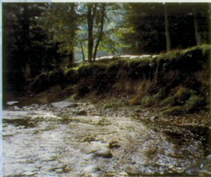
16. Erosion occurred on this site partly because trees and shrubs growing on an island to the left of the photograph were unmanaged and channel capacity was reduced. Coppicing some of the bankside trees will allow more light to reach the ground and reduce the weight on the top of the bank.
