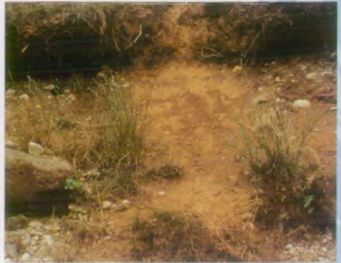
11. Damage to a riverbank may be exacerbated by too many people.
