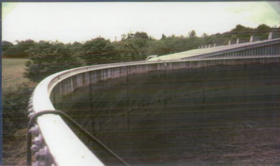
PHOTOGRAPH 1. Slurry Storage Tank at Westerhope Farm Showing the Fall in Level Associated with the Discharge.
