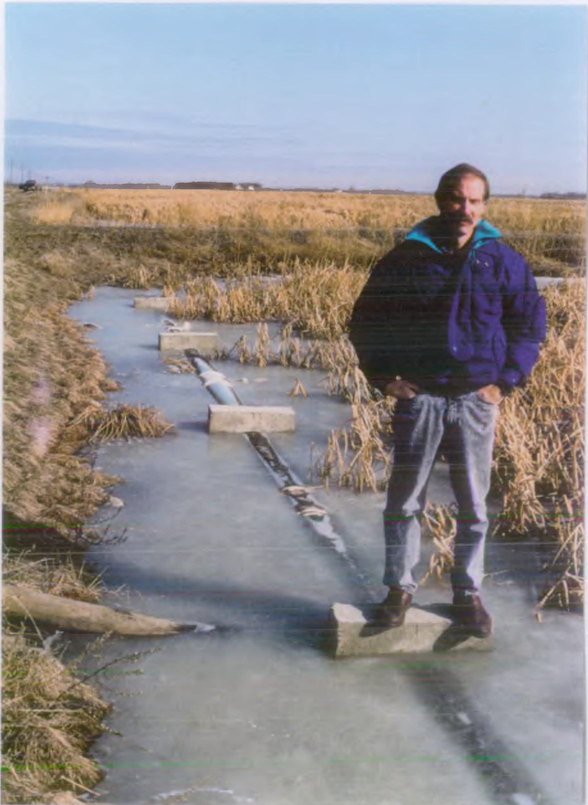
Water distribution system at American Crystal Sugar Corporation's Wetland Project.
