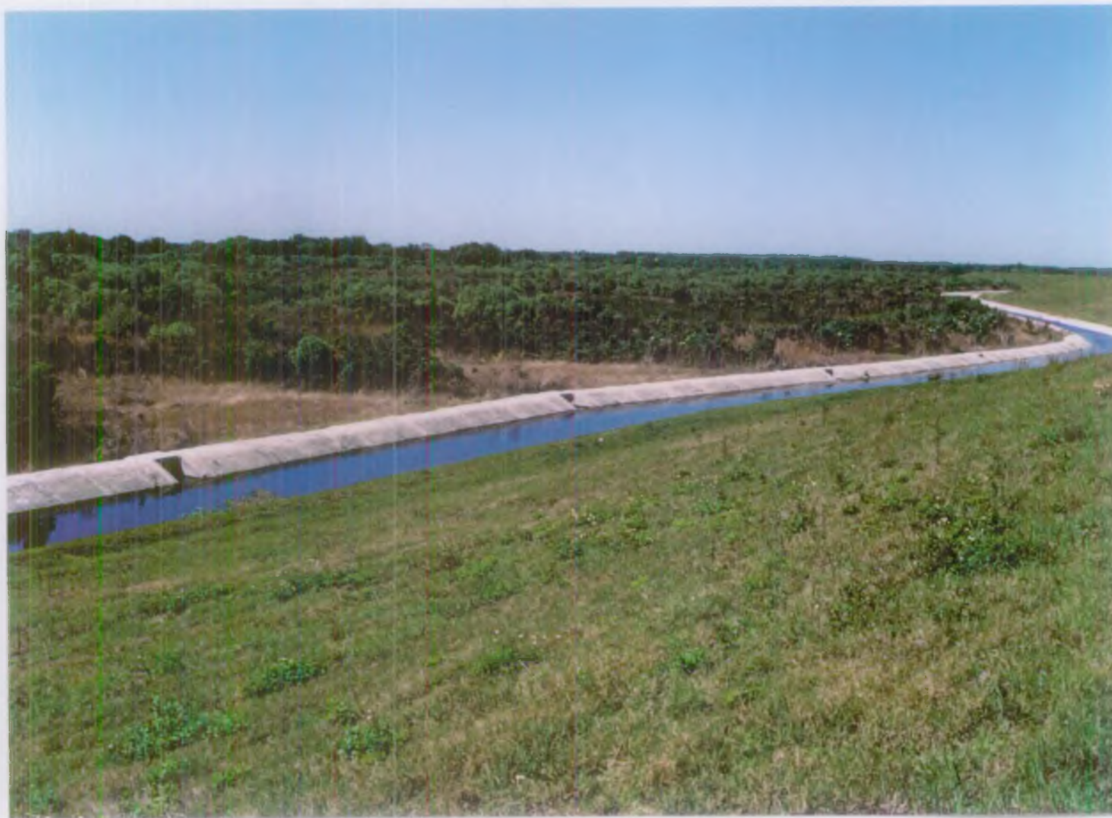
Water distribution system at City of Lakeland Wetlands Project.
