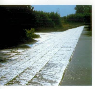
At Kegworth the "Shallow Lock" was lowered and a new "Deep Lock" was constructed to replace the existing deep lock. In the latter case, British Waterways funded and constructed the approaches to the new lock. Both the river and canal bridges were underpinned, the channel regraded between Kegworth Bridge and Kegworth Weirs and the length of the main weir was increased by 35 metres.
