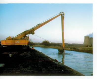
At Ratcliffe-on-Soar earth embankments approximately 1.5 metres (4.9 feet) high have been constructed alongside the village boundary to prevent the frequent flooding of the village. Landscaping including tree planting was incorporated into the scheme.
