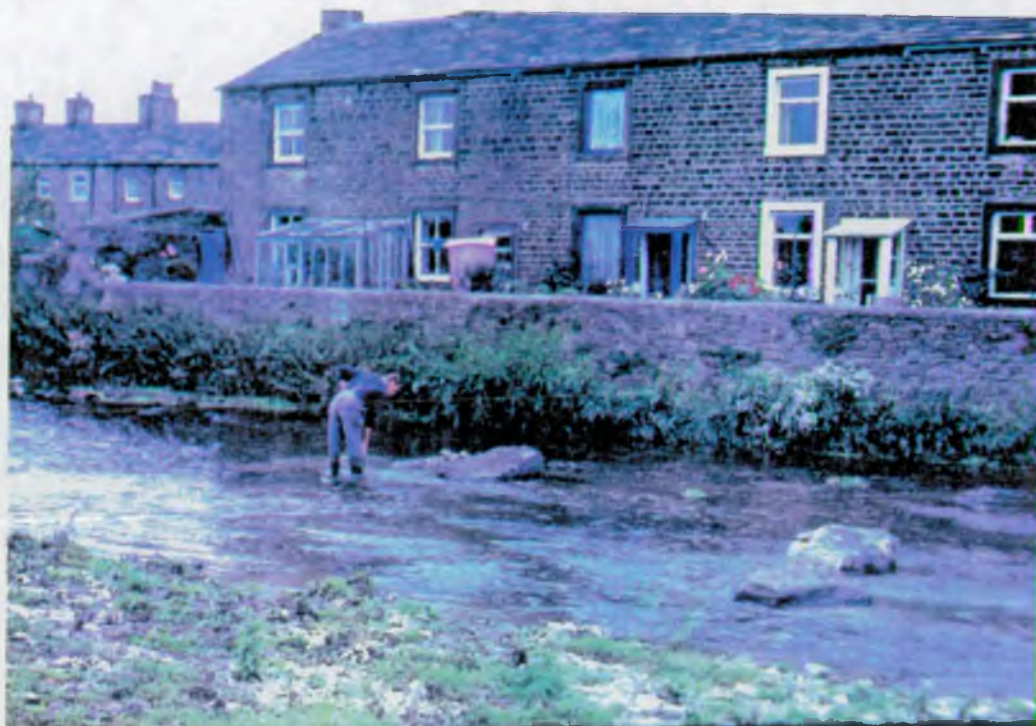
PHOTO 1 Introducing boulders to the River Aire at Gargrave to diversify fish habitats.
