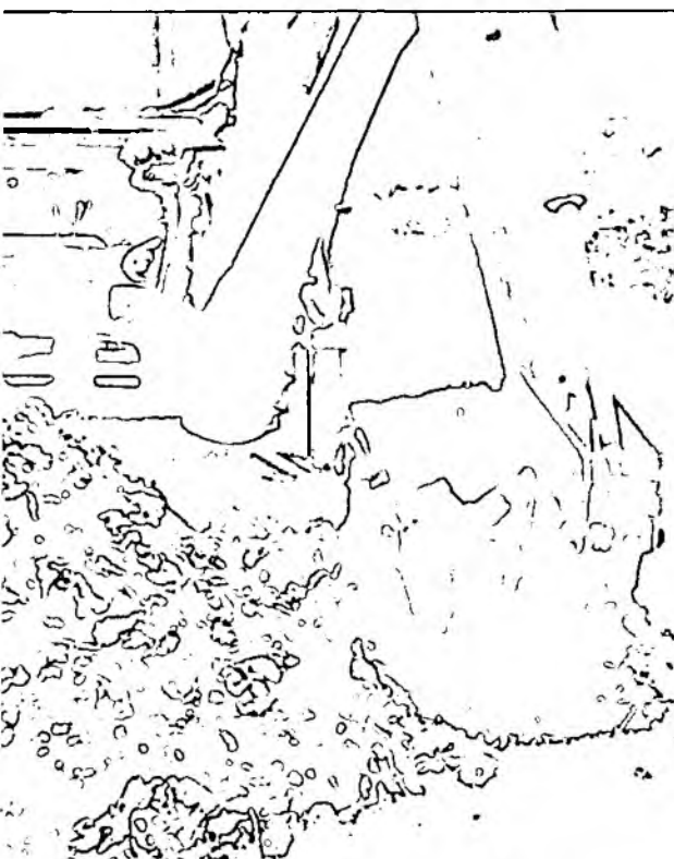
Trial pit investigation at a contaminated land site
