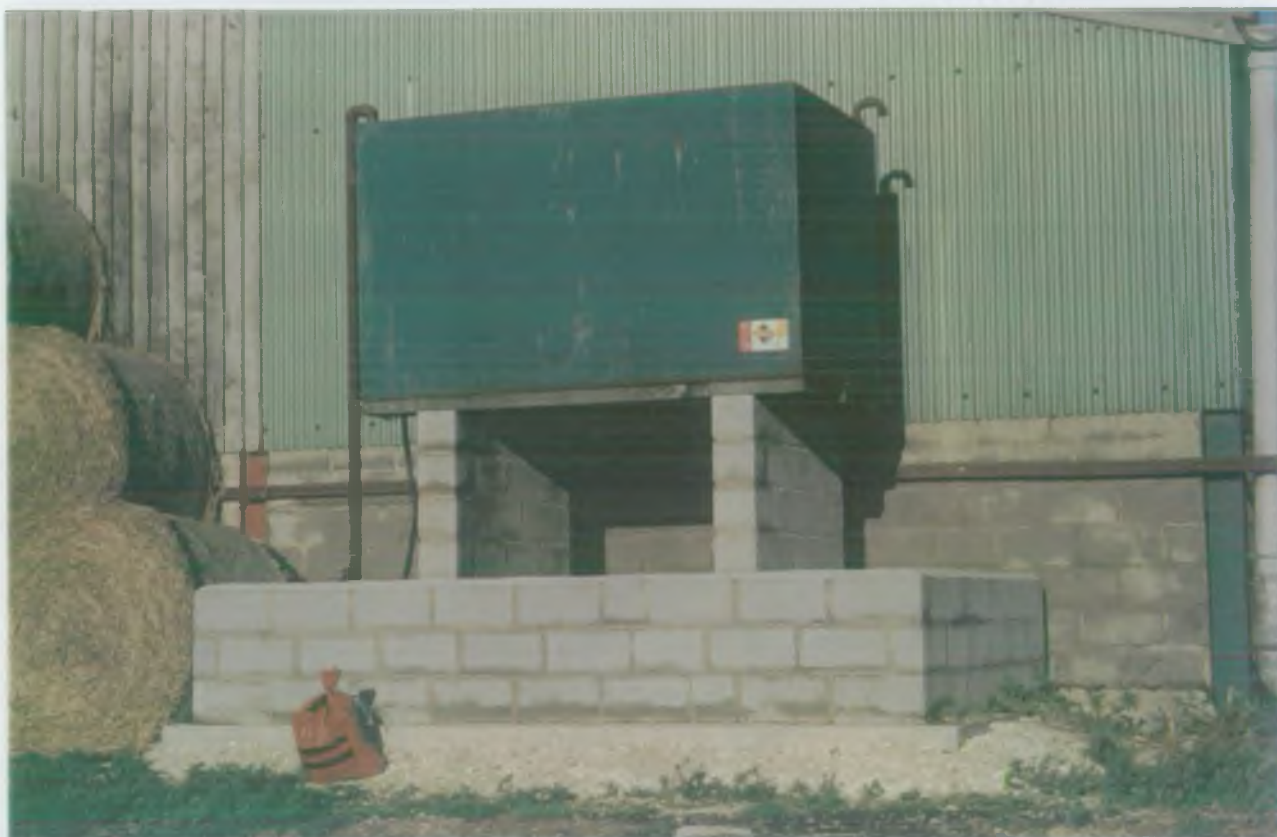
Farm oil storage tank bunded as a result of the Yorkshire Wolds initiative, North East Region See Section 3.5.8
