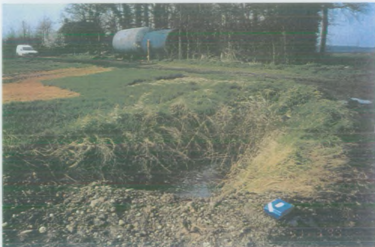
Liquid fertilizer tank with course of spillage shown by scorched vegetation, Anglian Region. See Section 2.1.1
