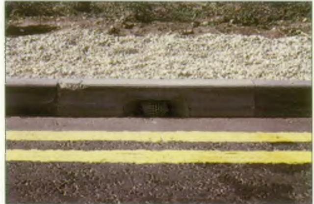
*Infiltration trench at the edge of a minor road. Water is taken into the trench via off-let kerbs.*
