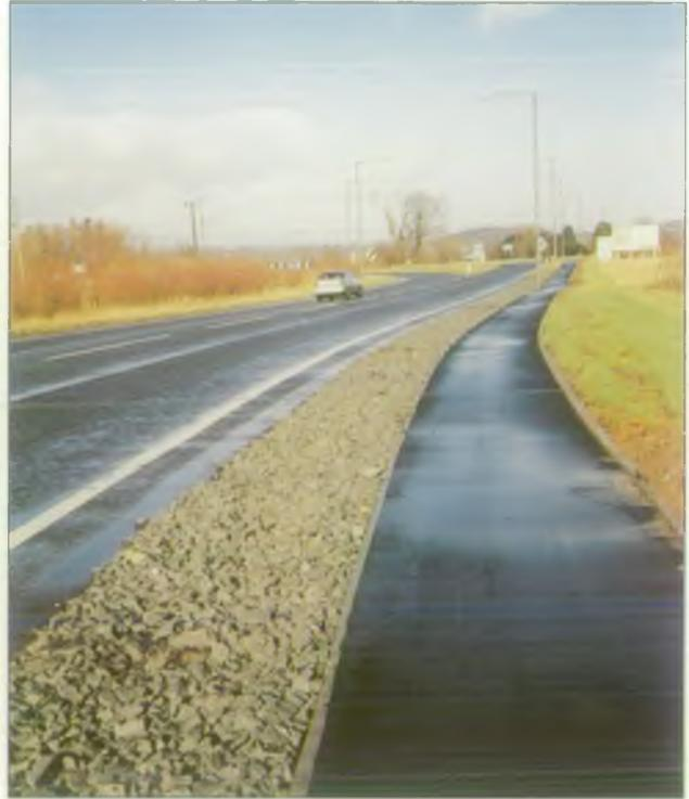
*A filter drain at the edge of a road in Stirling. There are no kerbs or gullies incorporated into the design.*
