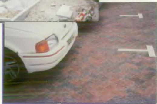
*Car parks with impervious surfaces are a common feature in the urban environment. Porous paving can be used to reduce the impact of car parks on flooding and water quality, without compromising the car park's utility. The design and construction of porous surfaces must be in accordance with the manufacturer's specification.*
