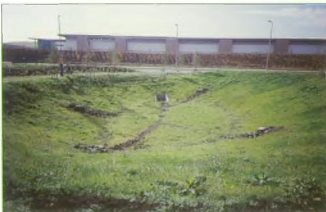
*Highway junctions provide land between slip roads that can be used for ponds or wetlands. In this case, land in the centre of a roundabout has been used as a detention basin, which releases rainwater at a fixed maximum rate, providing storage at times of intense rainfall.*
