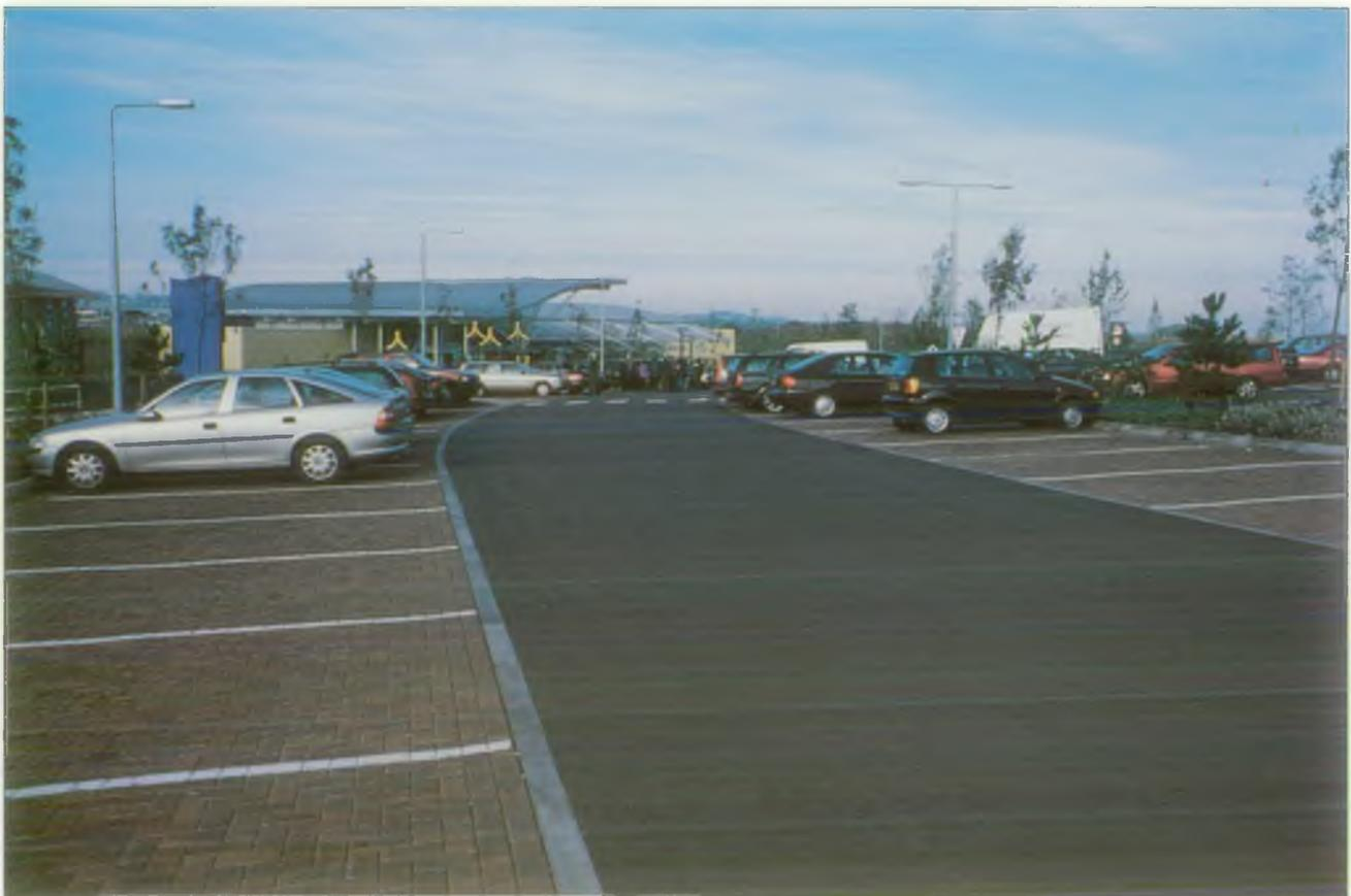
*Here the parking area at a motorway service has been built with porous blocks for the parking bays. The rainfall from the tarmac access roads runs onto these bays.*
