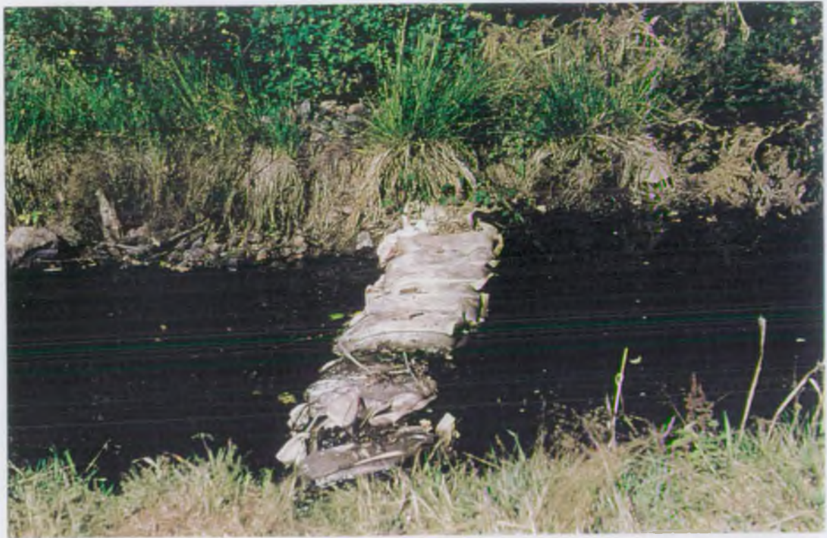
Plate 3 - Temporary sandbag weir at Crowndale Farm
