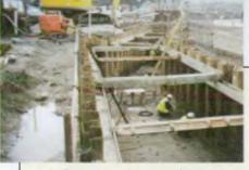
▲ Construction of the base of the combined inlet structure
