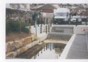
The completed combined inlet structure with angled screens (pipe to old outfall in centre, new culvert entrance under screen on right).
