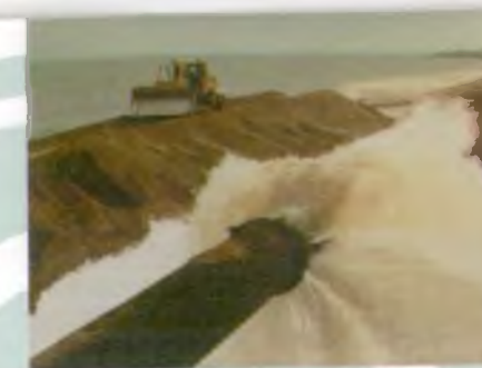
Sand and Shingle pumped ashore during beach nourishment
