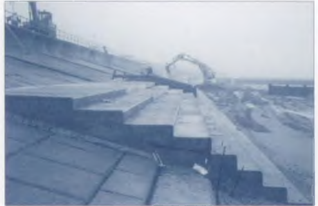
Stepped sea wall during construction
