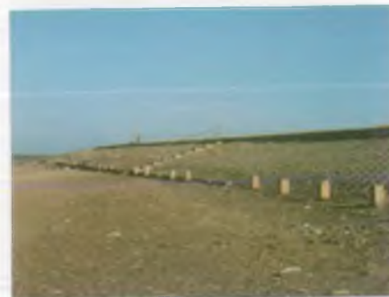
Heacham North Beach – Strengthened only with concrete revetment
