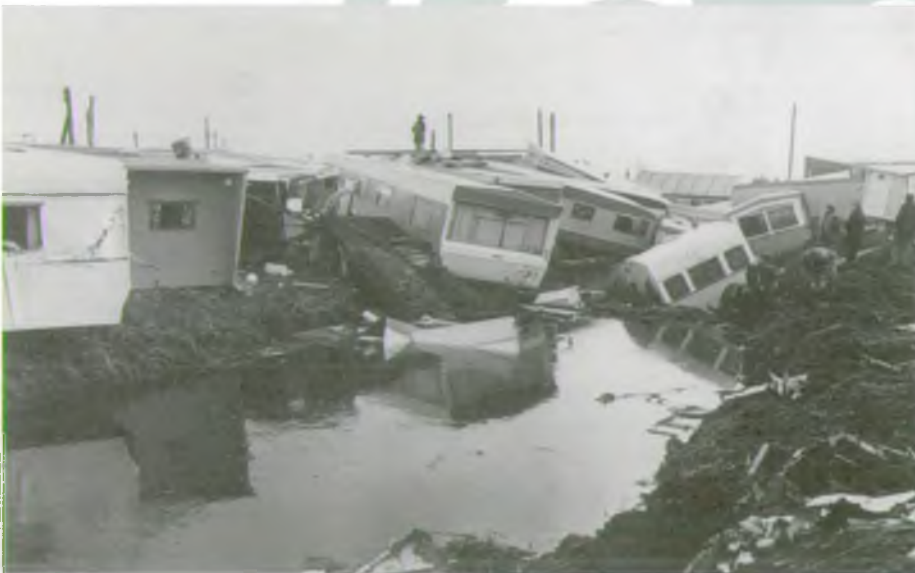
Damage caused by breach of sea defences at Heacham in 1978
