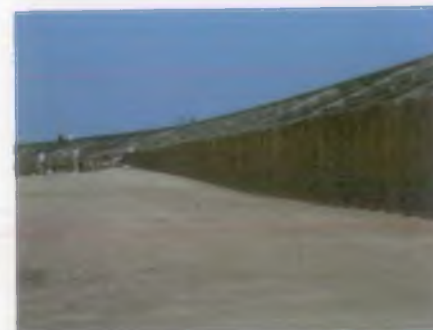
Hunstanton – as the beach levels reduce the toe piles are exposed
