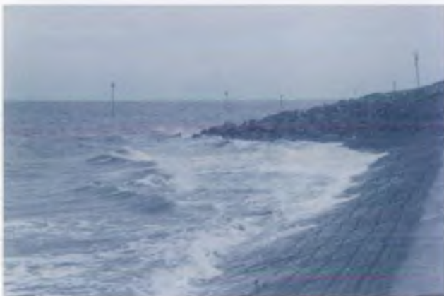
Existing concrete revetment at the site of the proposed works
