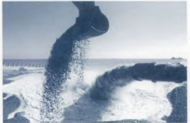
Nourishment works showing pipeline discharge
