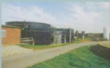
Davidstow Creamery treatment works
