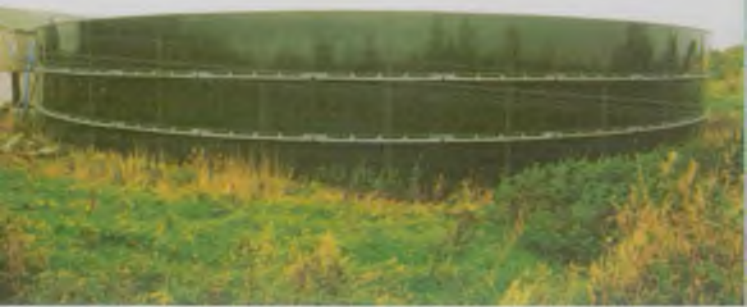
Circular slurry tank
