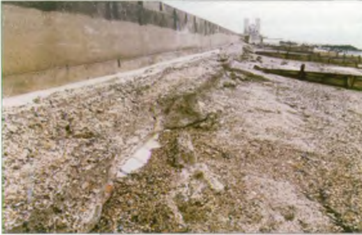
Reculver prior to works
