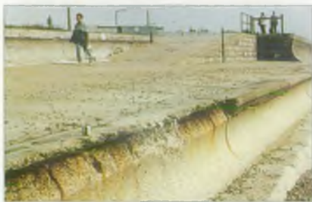
Dymchurch sea wall prior to improvement
