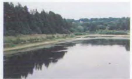
Dowdeswell Water will work in tandem with the part-time storage area at Cox's Meadow
