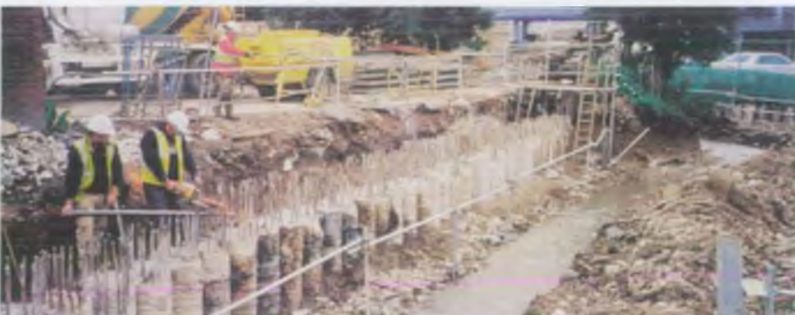
Work in progress during Phase 1
