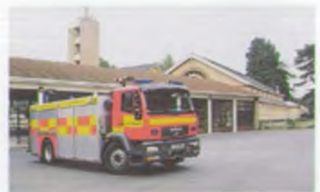
Cheltenham Fire Station headquarters
