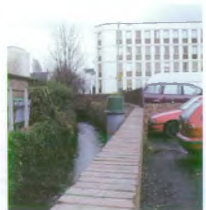
The culvert under Bath Road car park will be replaced with a wider one
