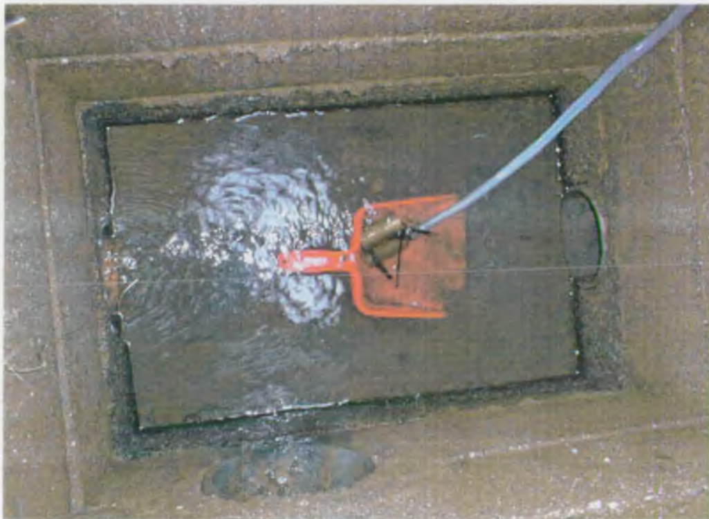
Showing view of sample tube in manhole.
