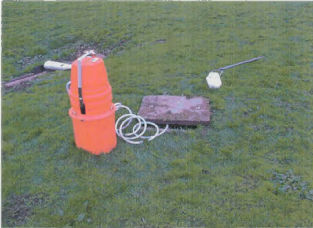
Epic auto-sampler next to manhole at site 7.
