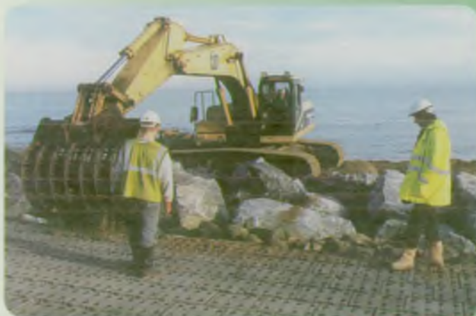
Rock armour is a frequently used method to protect the Anglian coastline
