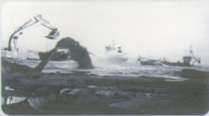
Slurry being pumped ashore
