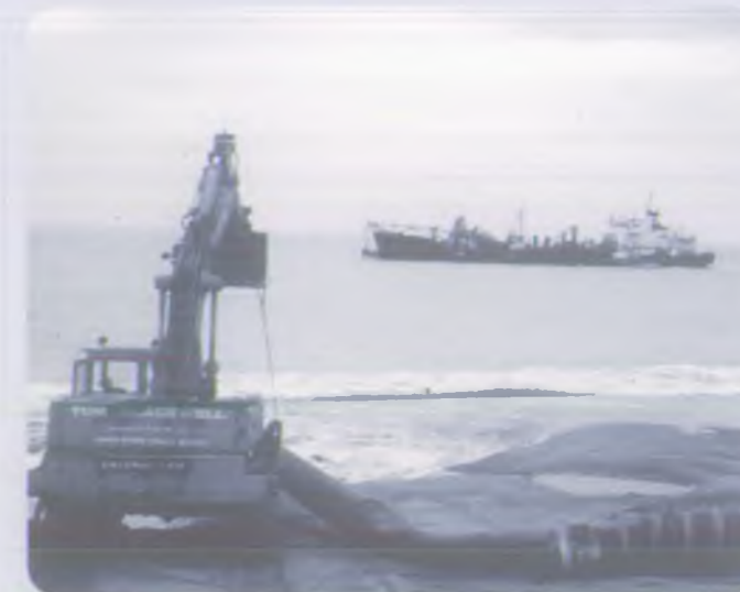
Material is screened before being pumped ashore
