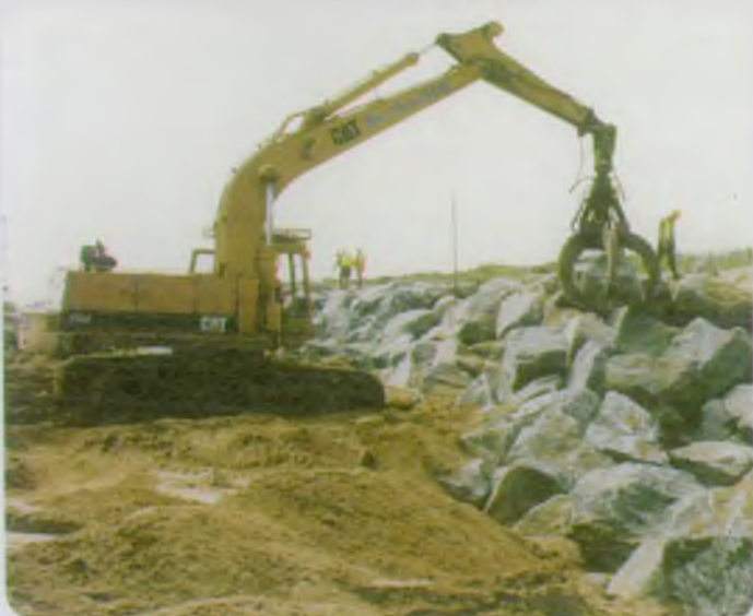
Work on hard defences at Skegness
