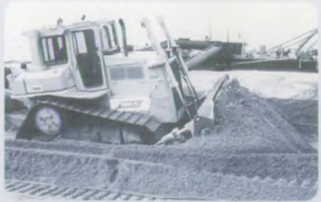
Earthmovers are in use throughout daylight hours
