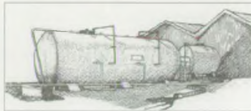
Unbanded storage tanks
