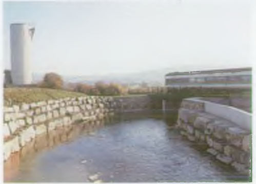
Channel realignment works - River Gronw.
