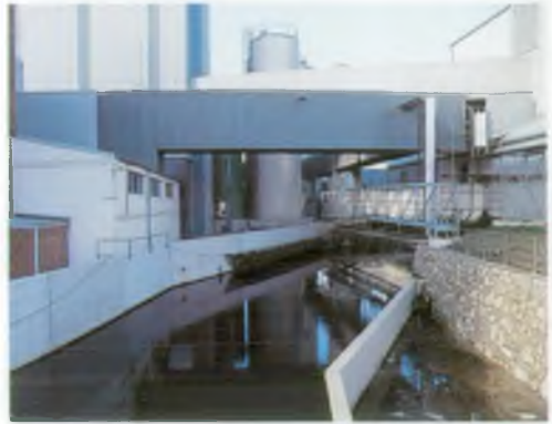
Side weir and sluice bypass channel.
