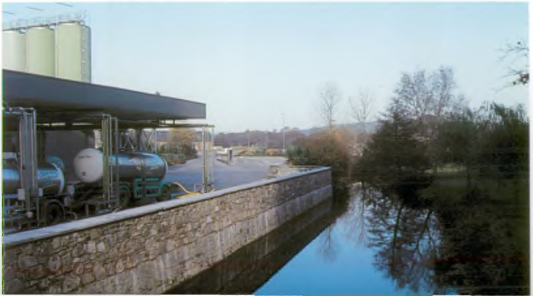
Side weir and sluice bypass channel.
