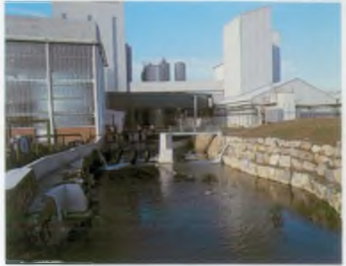
Realigned channel and flood defences upstream of railway bridge.
