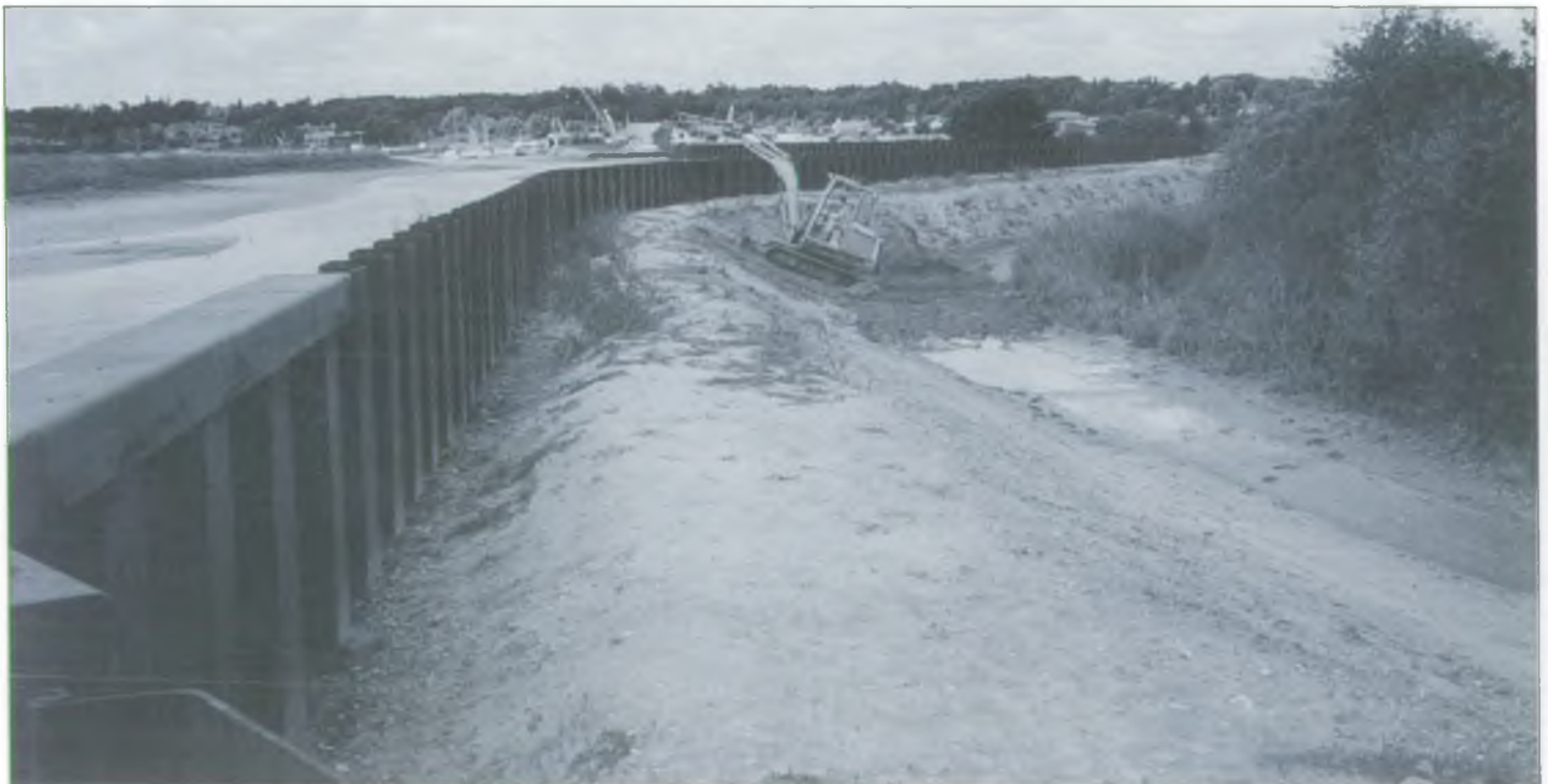
Below: New steel sheet piled defence, Melton Amenity Area.
