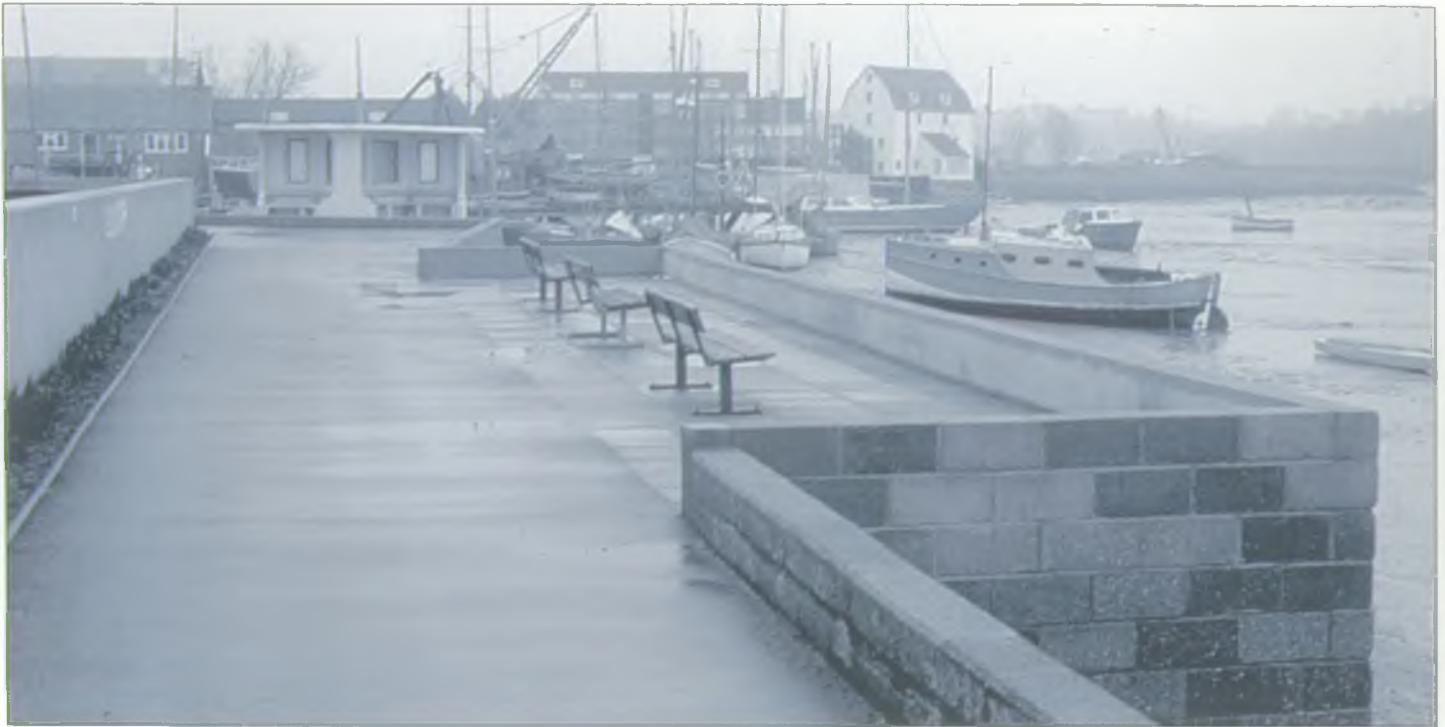
Above: Contract 2; improved seating area adjacent to new flood wall.
