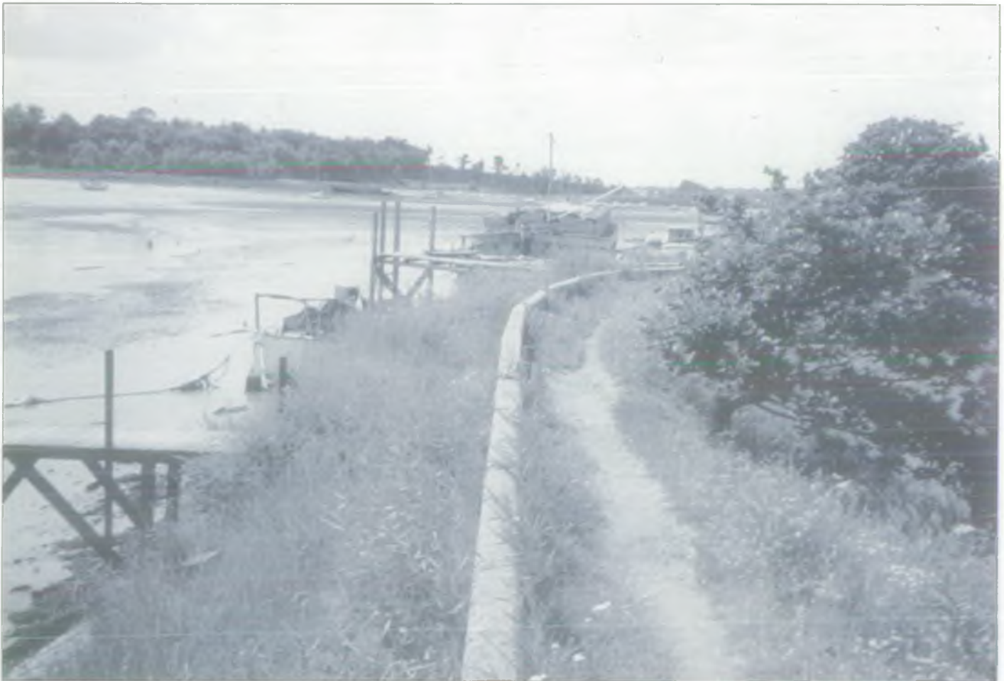
Above: Contract 5; Existing earth embankment and riverside footpath.
