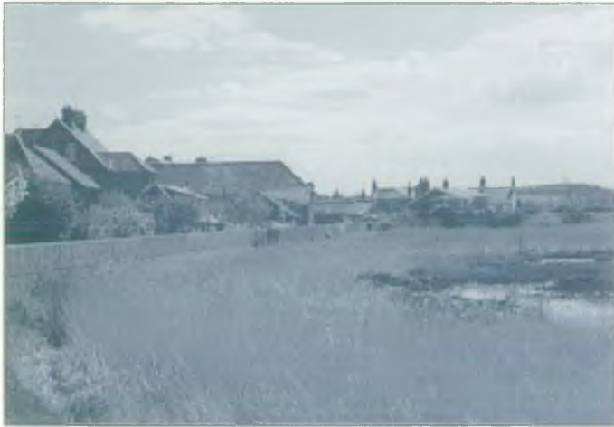
Existing town defence.
