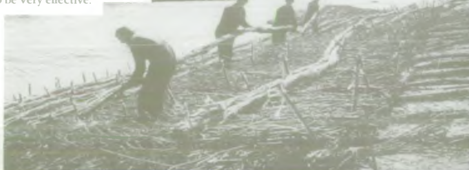
Laying a fascine mattress
