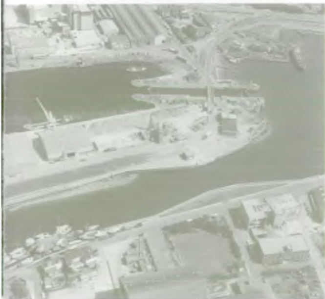
The River Gipping velocity control structure
