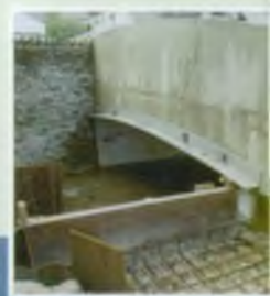
▲ Bridge under construction
