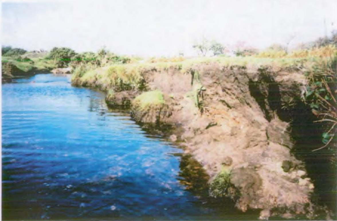
**Photo (14).** Area upstream of Dam 3 after breaching. Note the reduced water level. The effects of bankside undercutting can now be seen.
