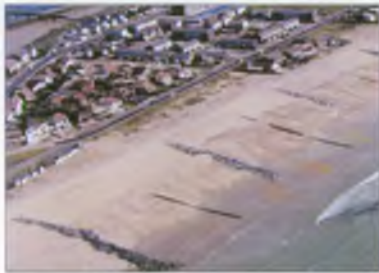
Rock groynes with beach recharge
