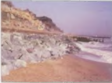
Scour protection to a seawall
