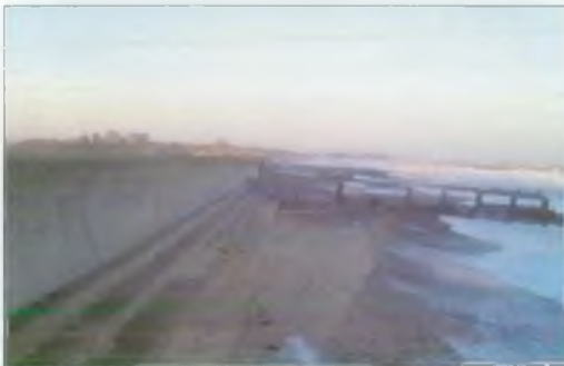
Short, closely spaced groynes appear to be more effective at retaining a beach than longer, more widely spaced groynes.
