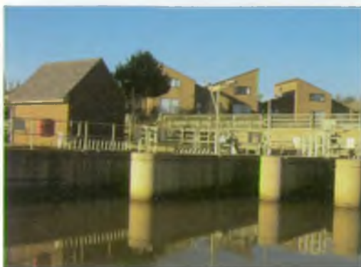
Eastern Yar sluices
