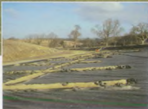
New landfill cell and drainage
