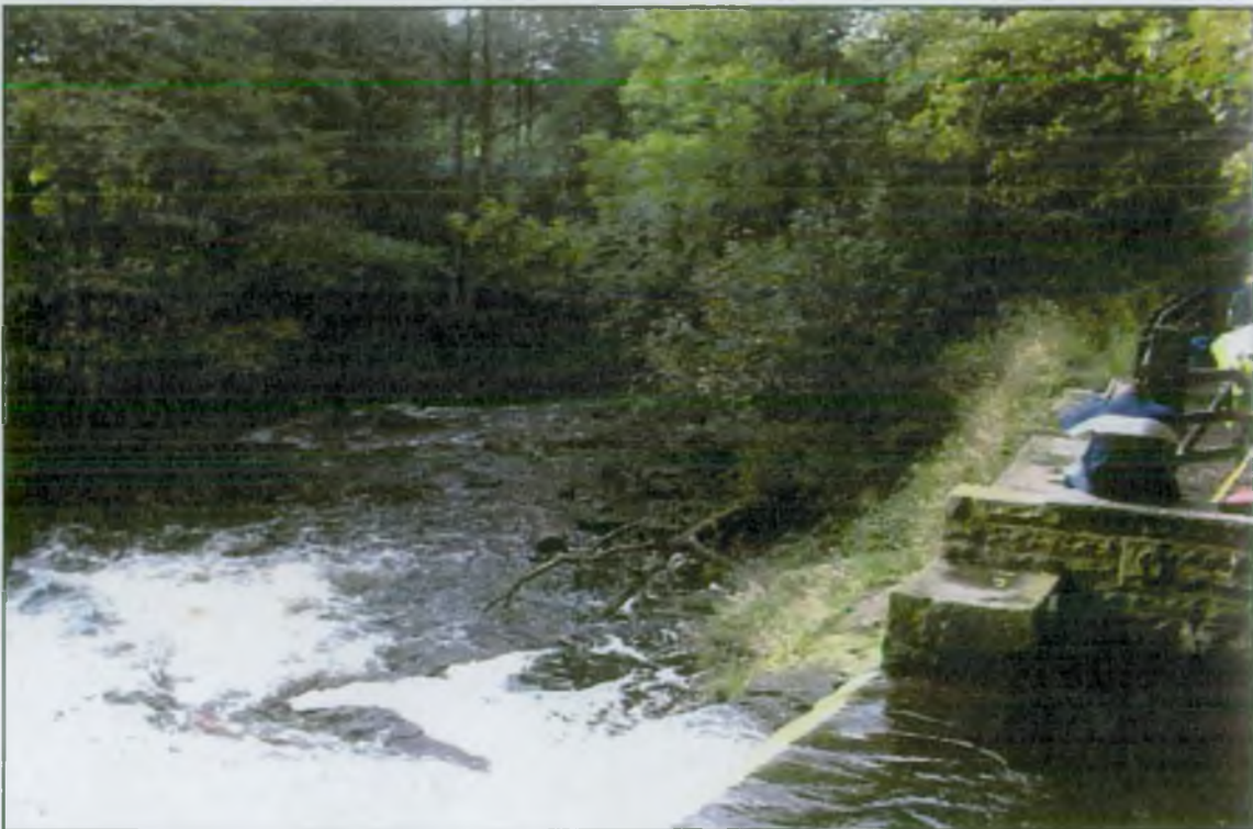
Cross Section – (YA100025) Looking Downstream
