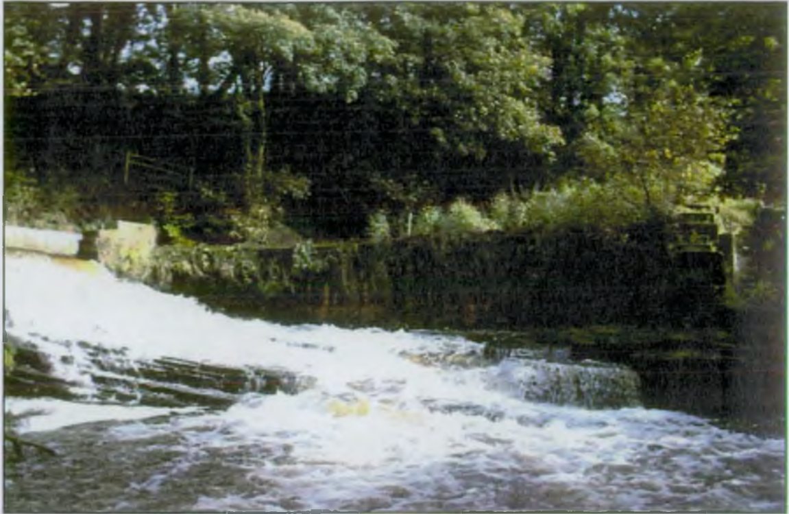
Cross Section – (YA100025) Looking Upstream
