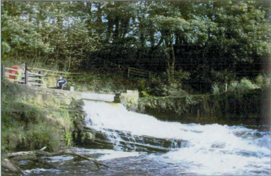
Cross Section – (YA100025) Looking Upstream
