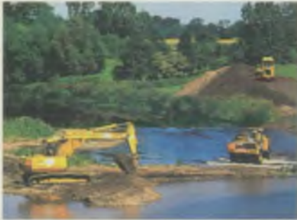
Flood defence works on the Tees
