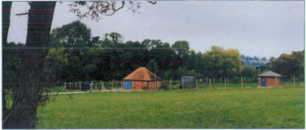
Right: Wellhead Pumping Station
