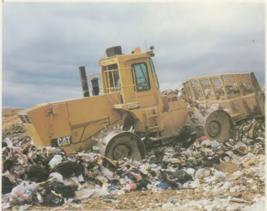
Work in progress at a waste disposal site
