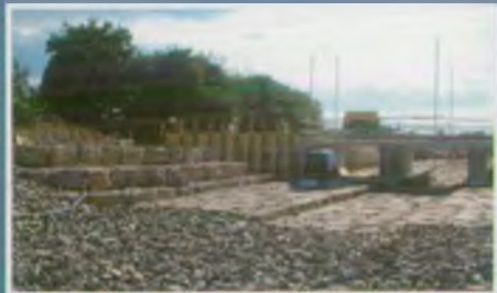
▲ New road bridge under construction
