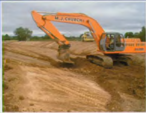
▲ Excavation of the main channel
