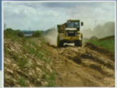
▲ Early earth works underway
