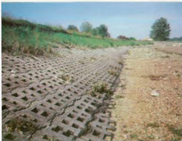
Example of concrete block revetment
