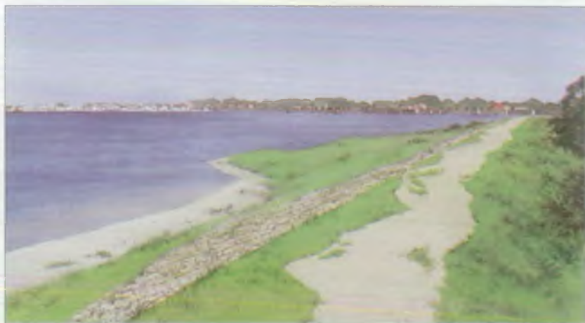
View of shoreline after embankment constructed
