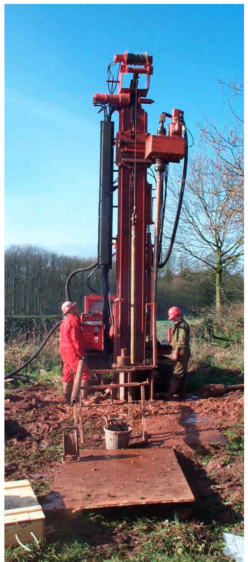
Drilling a monitoring borehole
