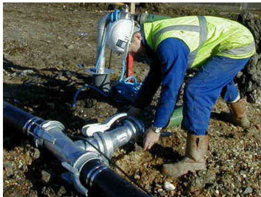
Photo A9.50 Connecting discharge pipe to deep wells
