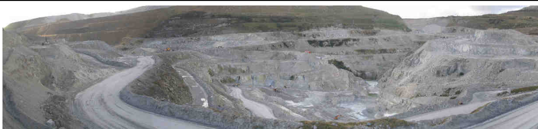
Photo A9.39 China clay excavation
