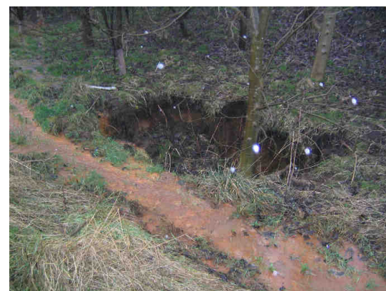
Photo A9.26 Sinkhole that appeared in December 2005
