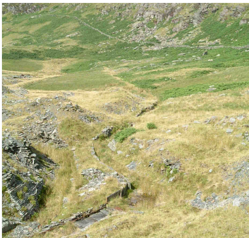
Photo A9.3 Old surface water drains
