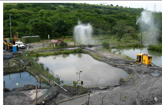
Photo A9.22 Vapour masts at stocking ground/railway loading area
