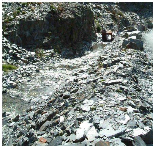
Photo A9.4 Surface water drain
