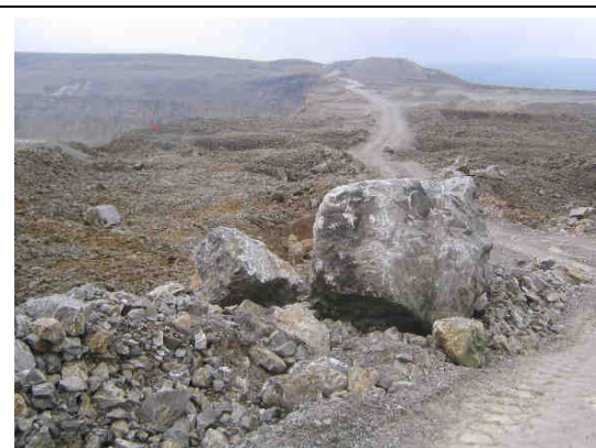
Photo A9.27 Overburden removed, showing surface of epikarst
