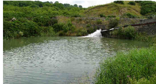
Photo A9.18 Settlement pond
