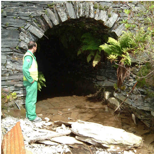
Photo A9.2 Adit discharge point
