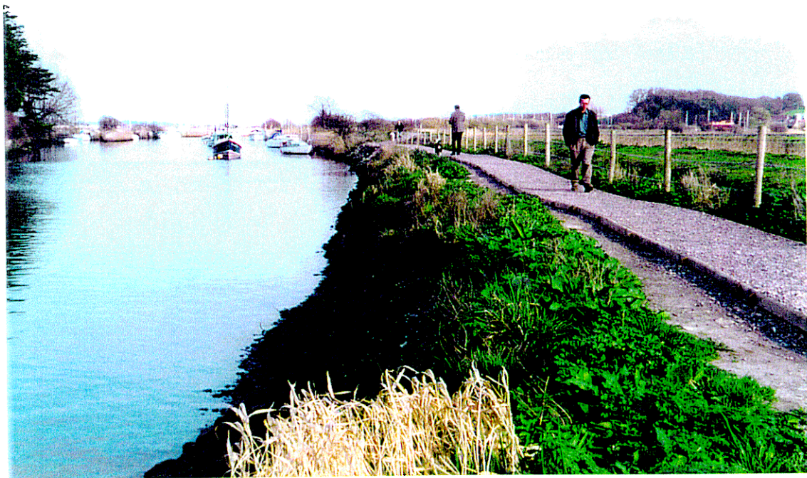
Plate 6 : New section of path adjacent to South Bridge, Wareham
