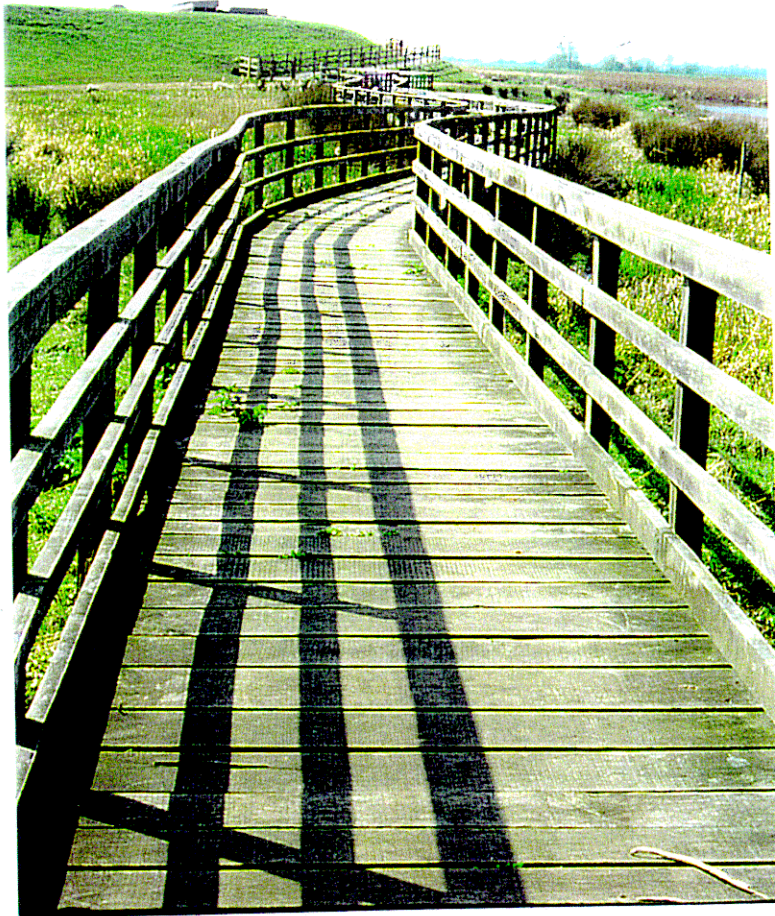
Plate 25 : Wooden board walks at Welches Dam used to prevent trampling of wetland vegetation, and allow wheelchair access
